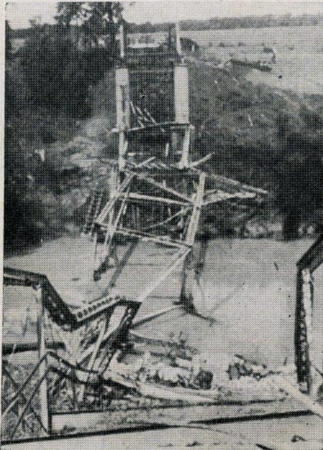
Navasota's Pat Griffith took this picture of the Navasota River Bridge after it fell. A truck load of men had passed over the bridge a few minutes before it collapsed.
