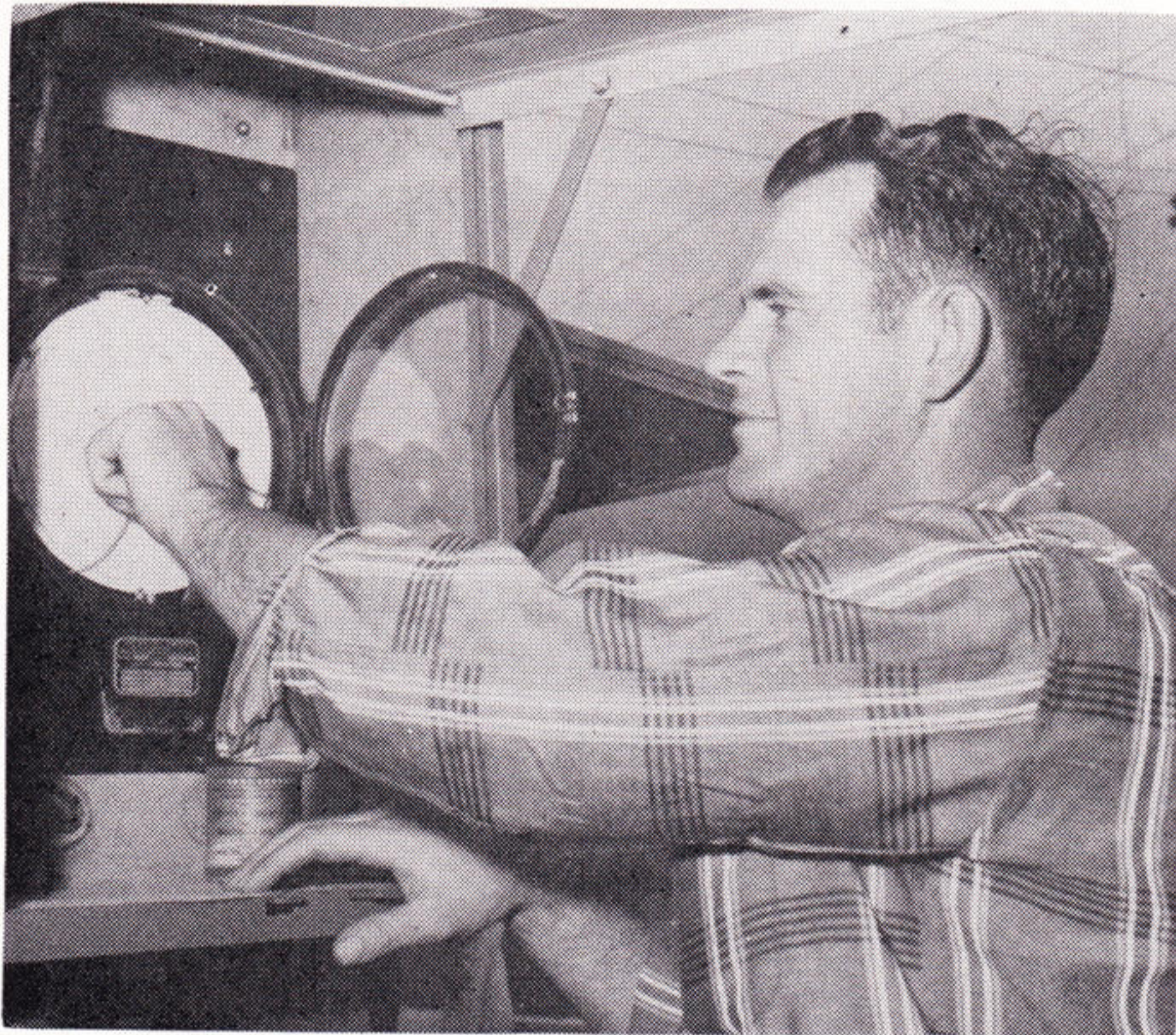
Daily duty — servicing substation meter.
