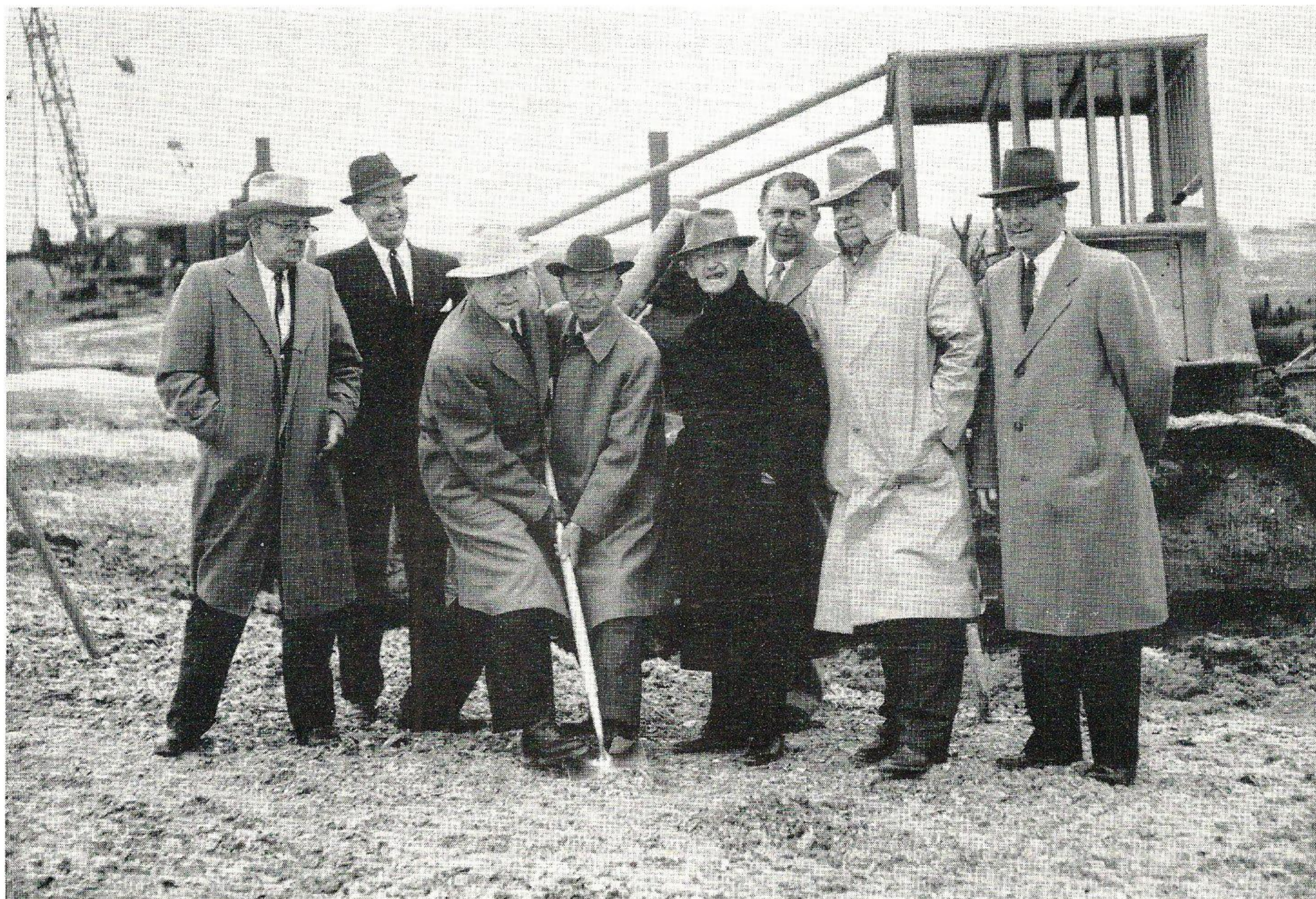
Roy S. Nelson, president and chairman of the board, gets a hand from Edgar Brown Jr., Orange businessman, in turning the first shovel of dirt at the groundbreaking ceremonies for the new Sabine Power Station. Representing West Orange; Howard Peterson; C. H. Meeks, mayor of Orange; Edgar Brown II; and T. O. "Doc" Charlton, district superintendent.
