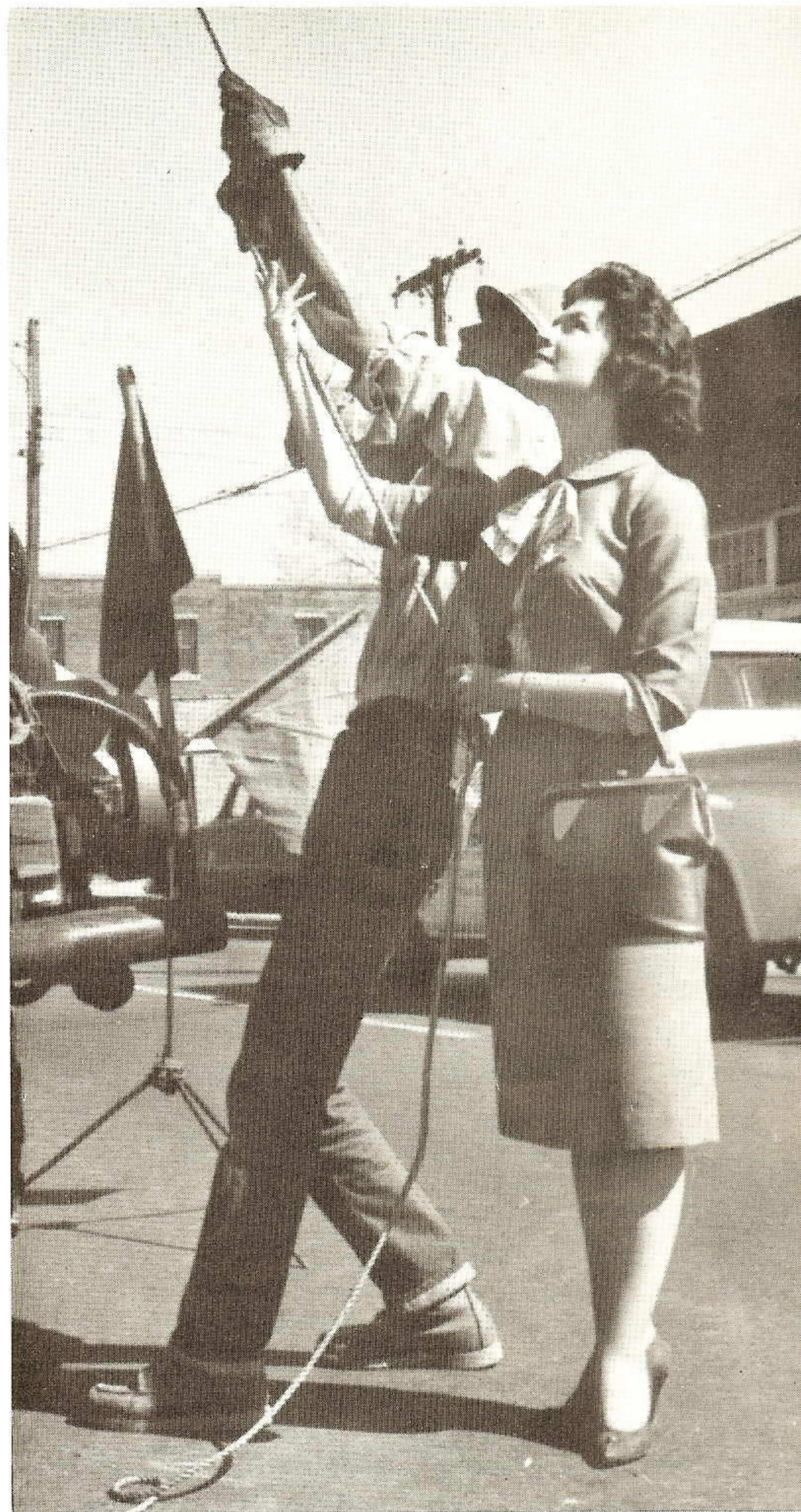
C AROLYN ST. AMANT, home service advisor in Baton Rouge Division, shows what the well-dressed grunt will wear. She and train Helper Elgin Caston are giving the old heave-ho to pull tools up to a lineman on the pole.
