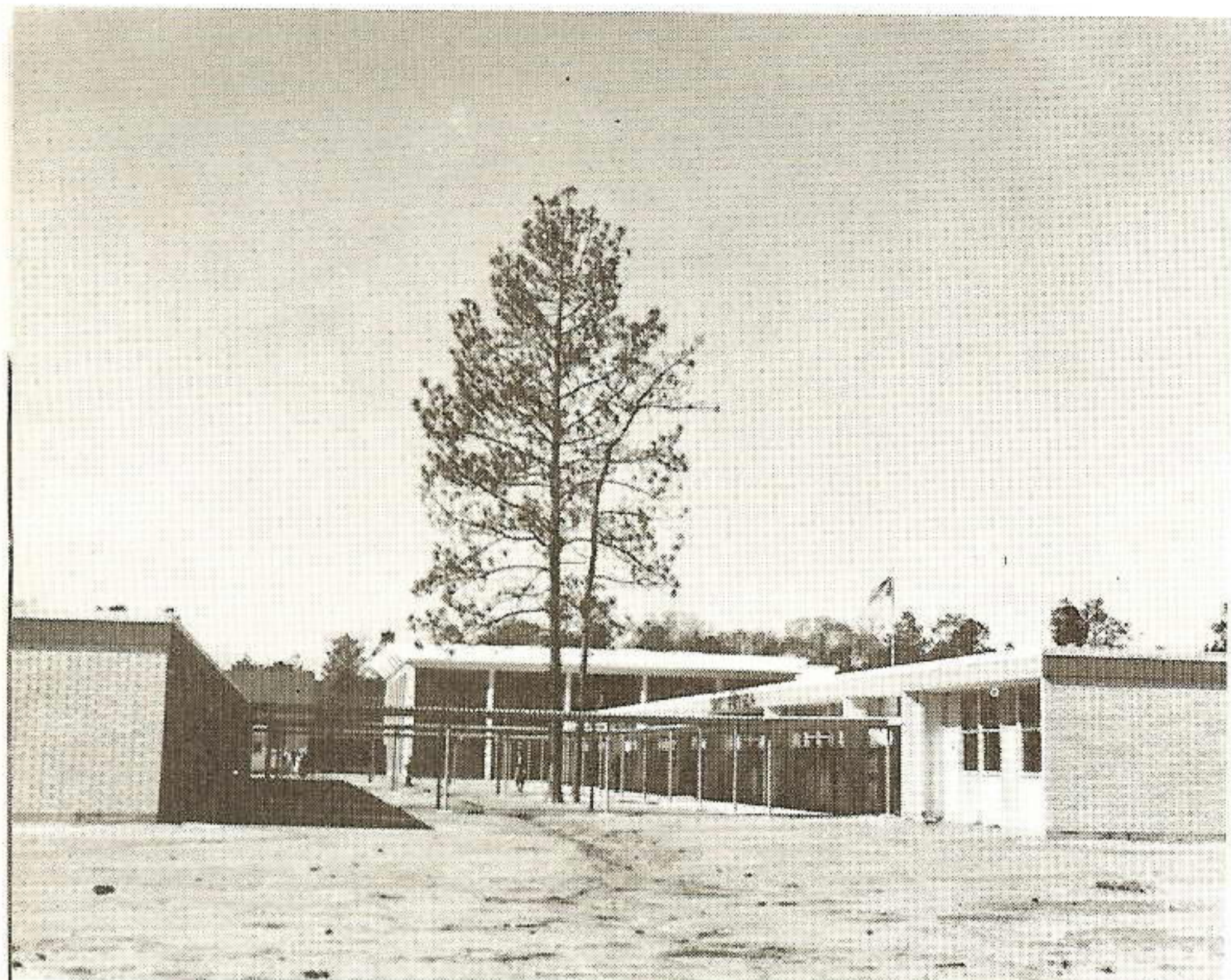
BEAUMONT DIVISION'S FIRST. Chance-Loeb's new school, occupied last November, is the first all-electric school constructed in the Beaumont Division. The new school features 24 individual class rooms, a spacious cafeteria, and the comforts of year 'round heating, air conditioning, and adequate defense lighting.
