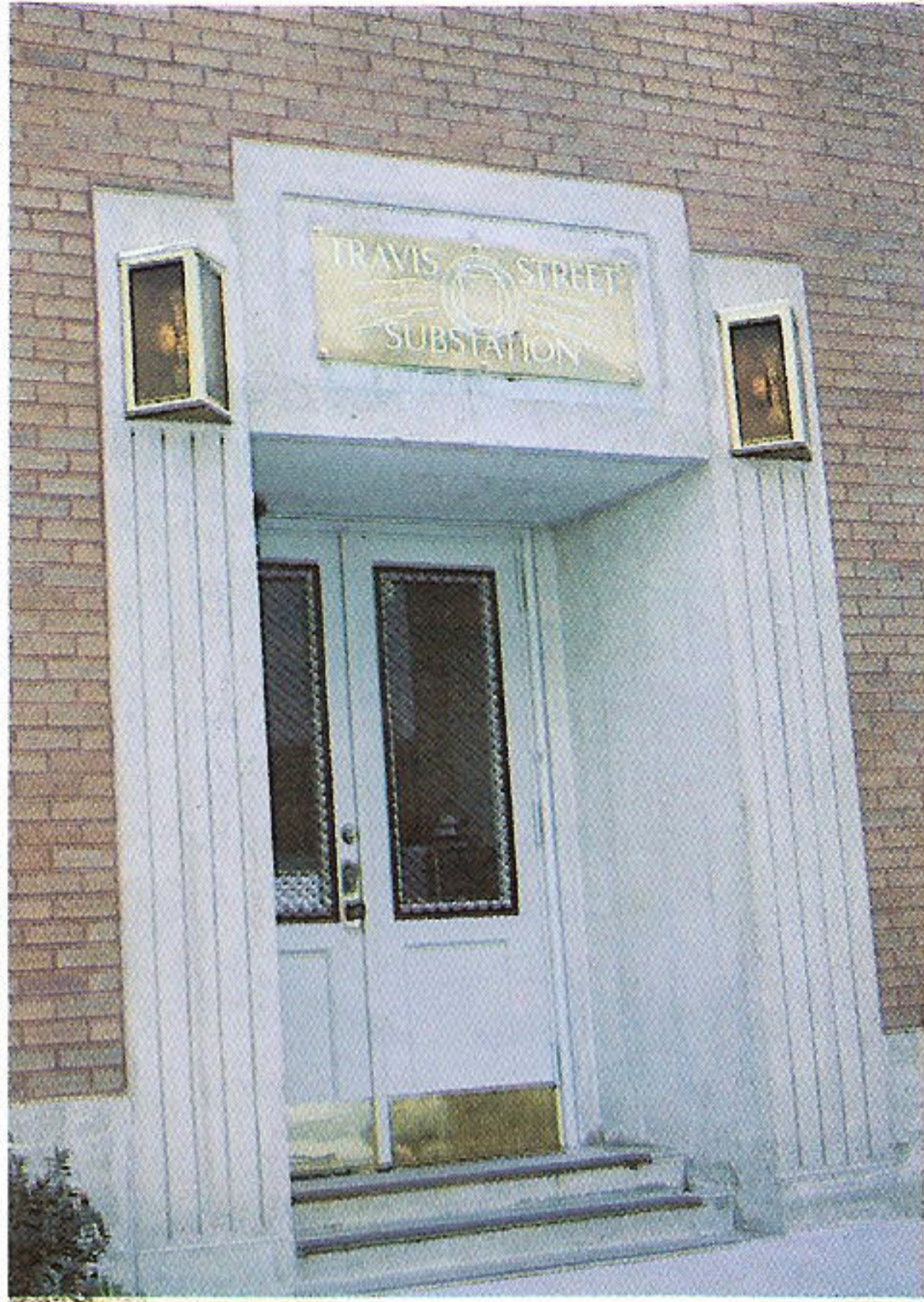
The former Travis Street Substation in Beaumont houses the only collection of Edison memorabilia west of the Mississippi.
