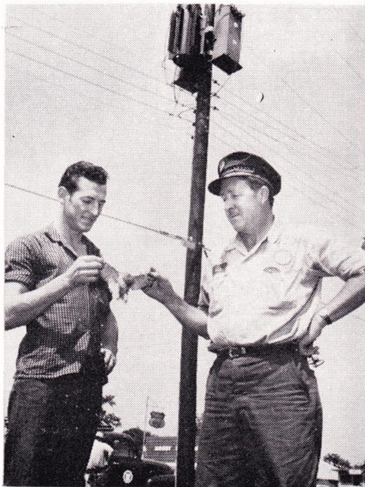
"Fried" bird was the result when this feathered fellow flew into one of our transformers. This transformer serves the First National Bank block in Cleveland. Gulf States crewmen are shown in the background restoring service which was interrupted by the "kami-kaze" bird.
