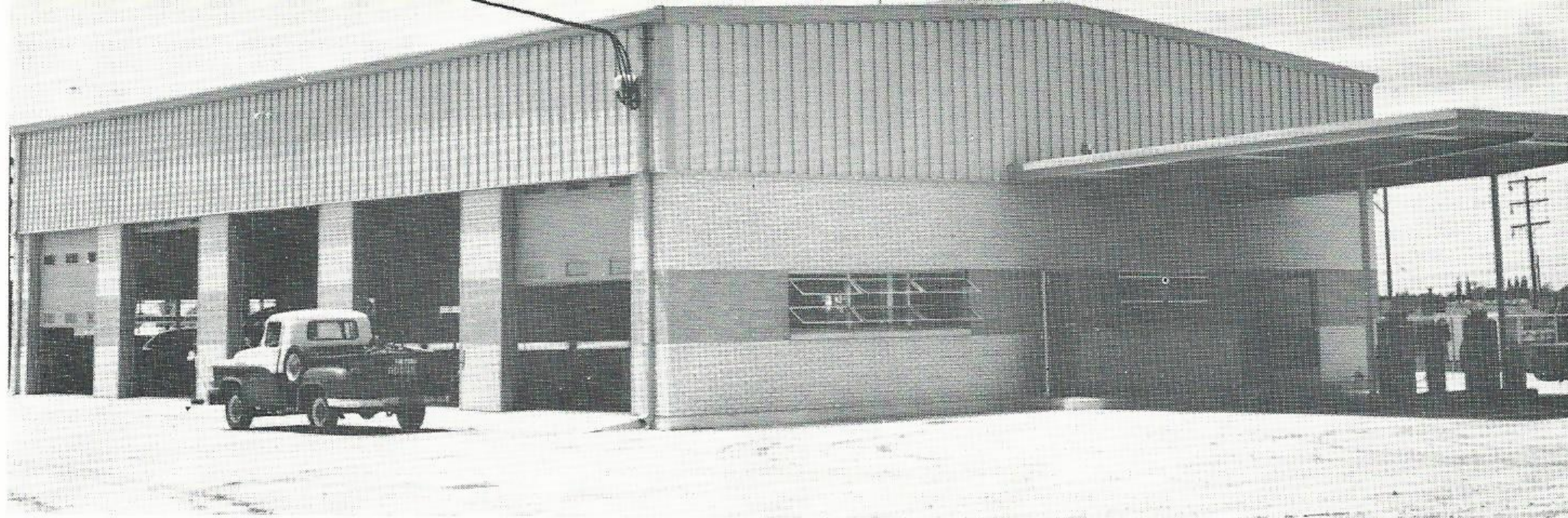
NEW NAVASOTA GARAGE. Employees of the Navasota Division garage moved into this modern service garage last month. The building is only one of three in the United States in which electric water heaters
