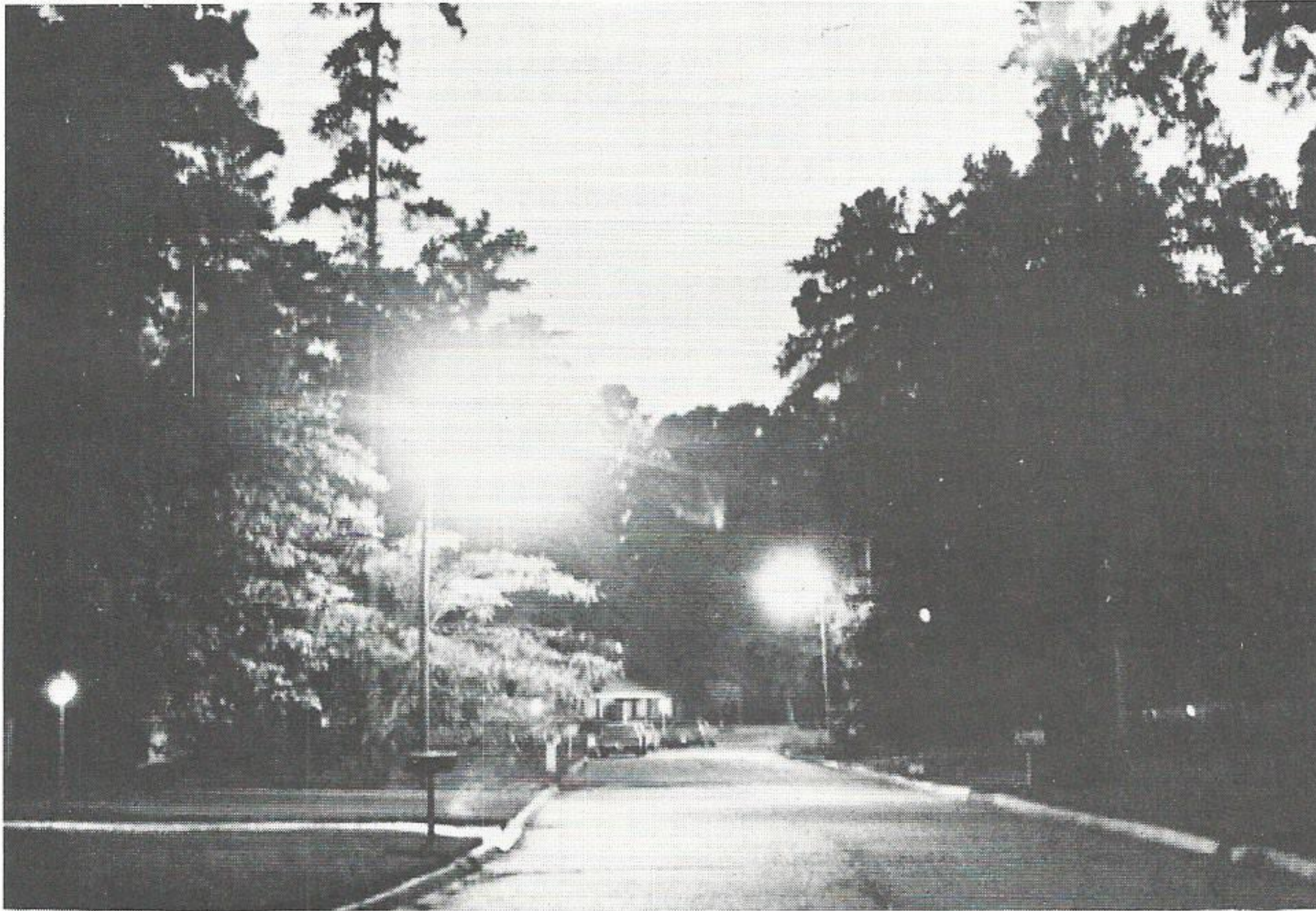
Wexford Park, laying just outside Vidor, Texas, sports a new look with its mercury vapor lights. The system was installed at the request of the residents, with each home owner paying a little each month.
