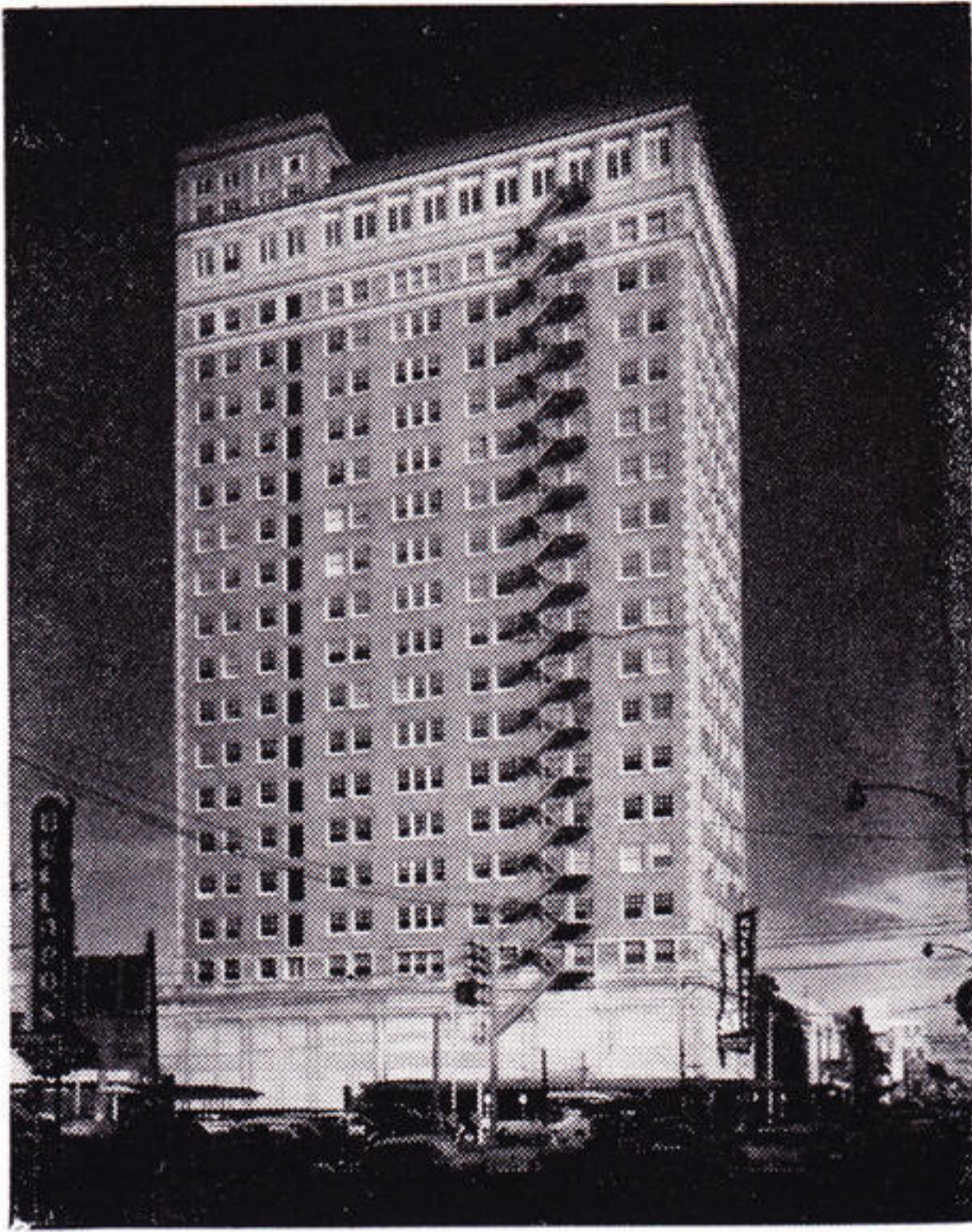
Establishment of our new Company headquarters in the 22-story general office building in Beaumont in August was another milestone in our history.
