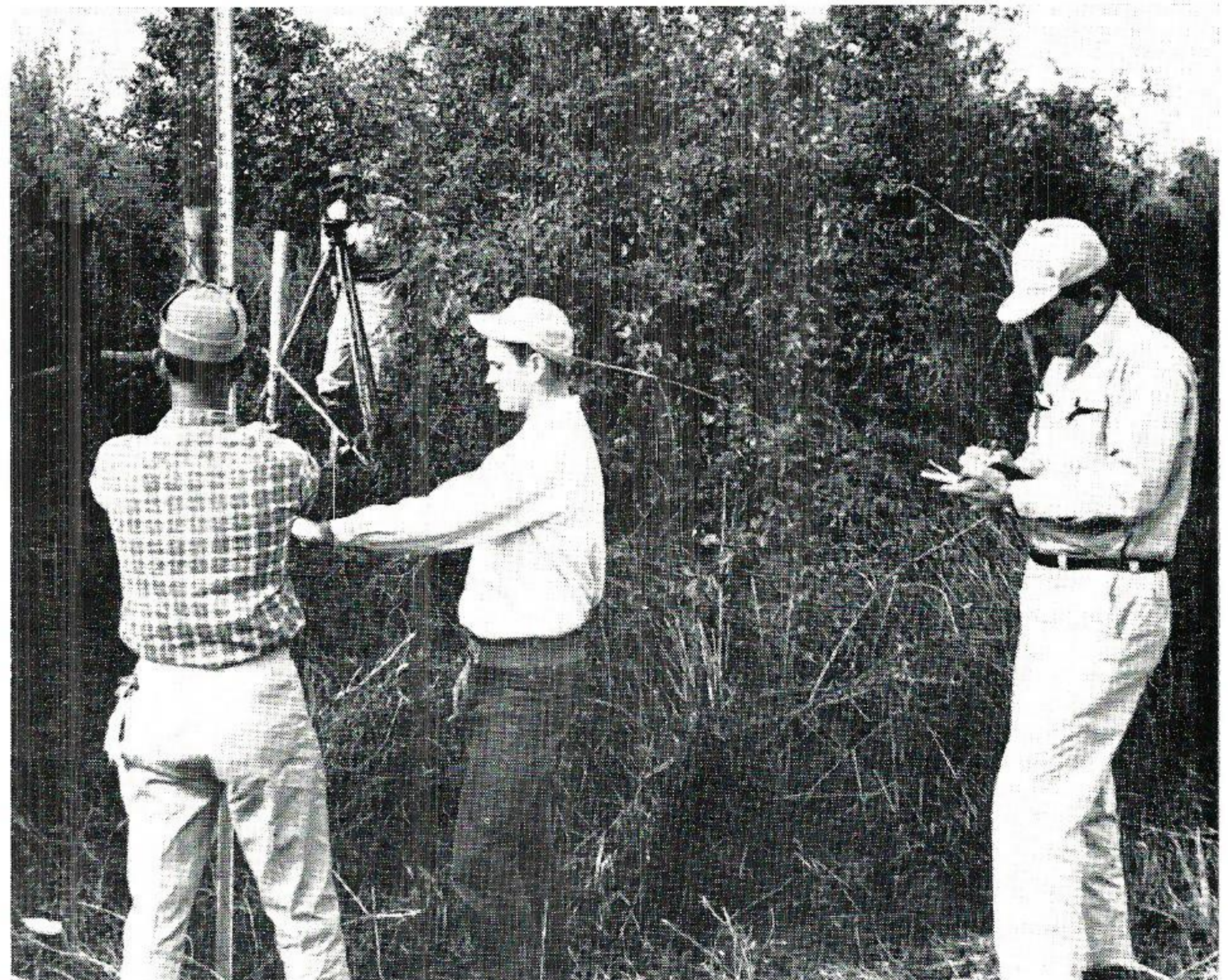
"TOPO" SURVEY. In the ditch are Messrs. Perolio and Coleman, holding the measuring stake as the instrument man sights on it.
