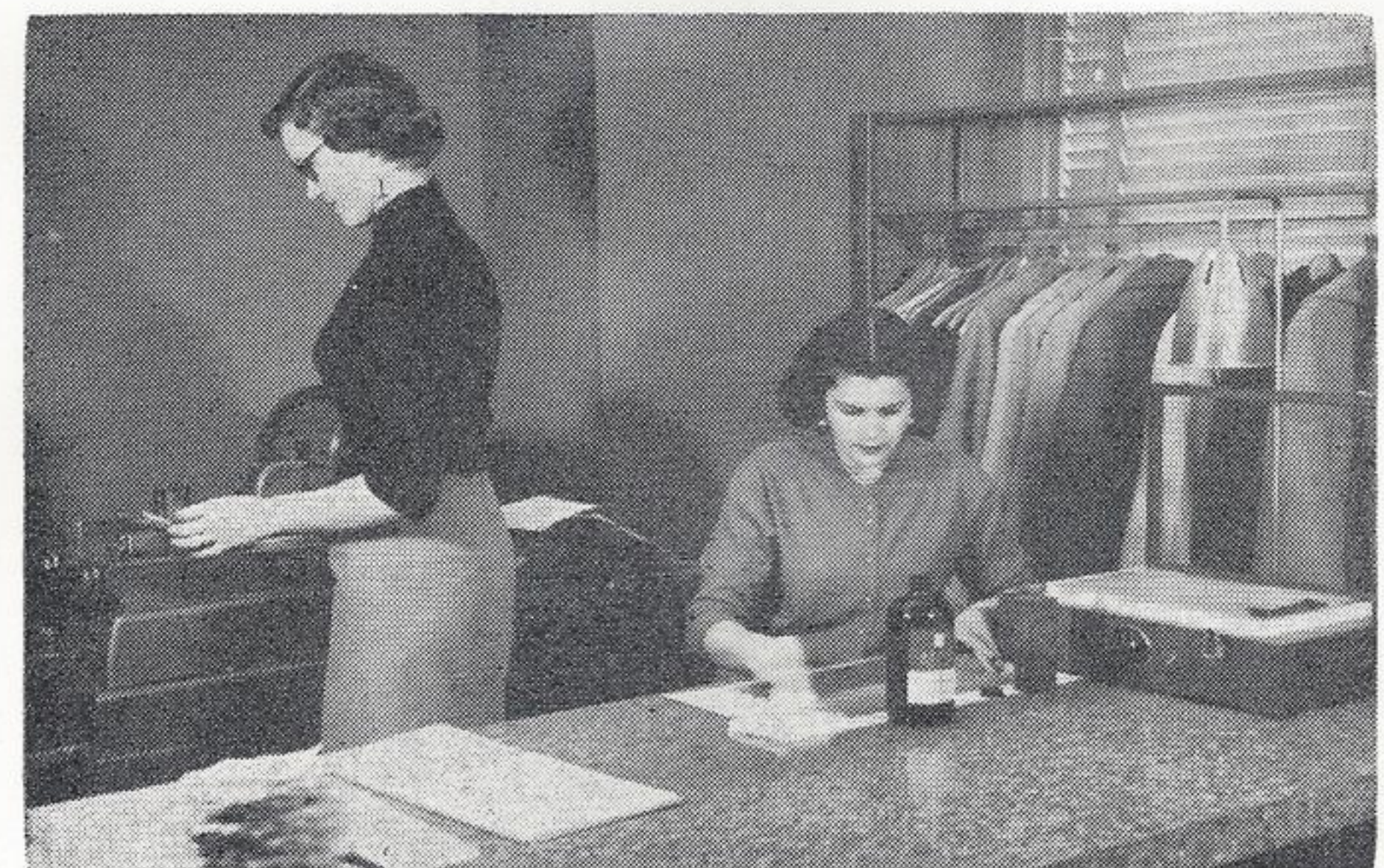
Gloria Bishop operates the mimeograph machine at left while Erline Cessac works at the exposure frame, which is used to make pre-sensitized masters from positive negatives. After the master is prepared, many copies can be run off swiftly and neatly.
