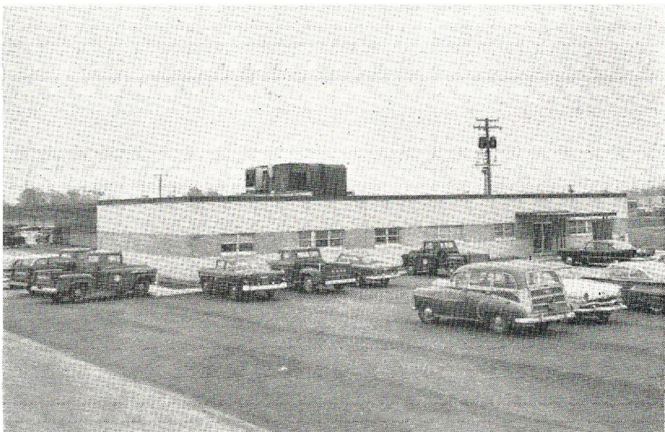
The new centrally-located Gas Service Center on Choctaw Drive in Baton Rouge provides the Gas Department with improved yard facilities, and the 15,000 square feet of floor space alleviates the crowded Government Street site formerly shared with the Electric Department.
