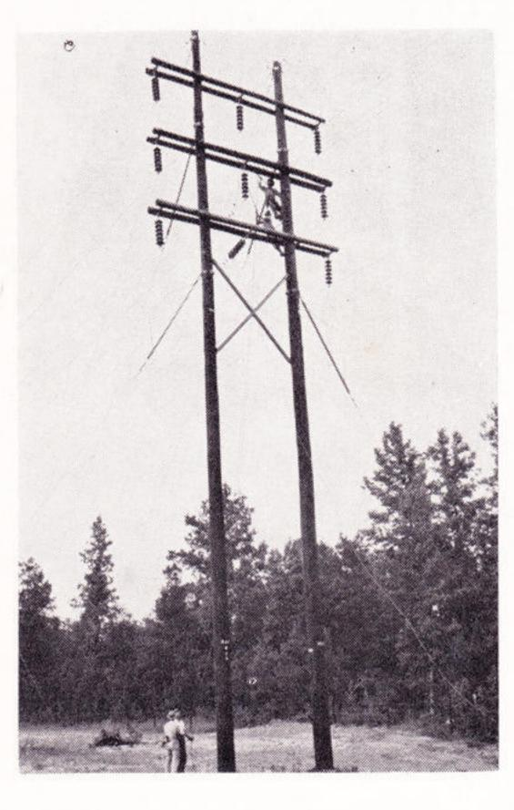
Lightning, like ice, is a hazard to power lines and causes expensive burn-downs. Lake Charles linemen (left) restore the 69 kv De Ridder lines after lightning damage. Part of a new 34.5 kv loop around Beaumont is the landscaped unit type Lawson substation (right).
