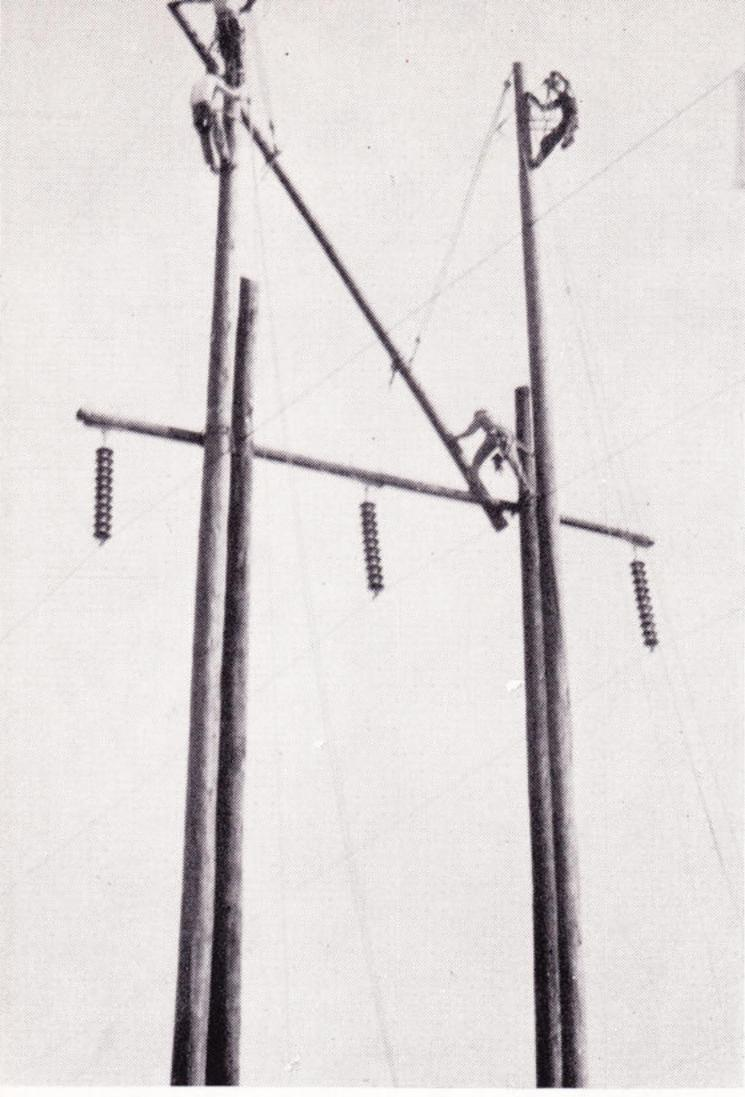
On the GSU-LP&L interconnection job, Linemen Stevens, Minor, Gordon and Baldin raise the 138 kv line almost 80 feet over the Port Allen No. 2 substation site.
