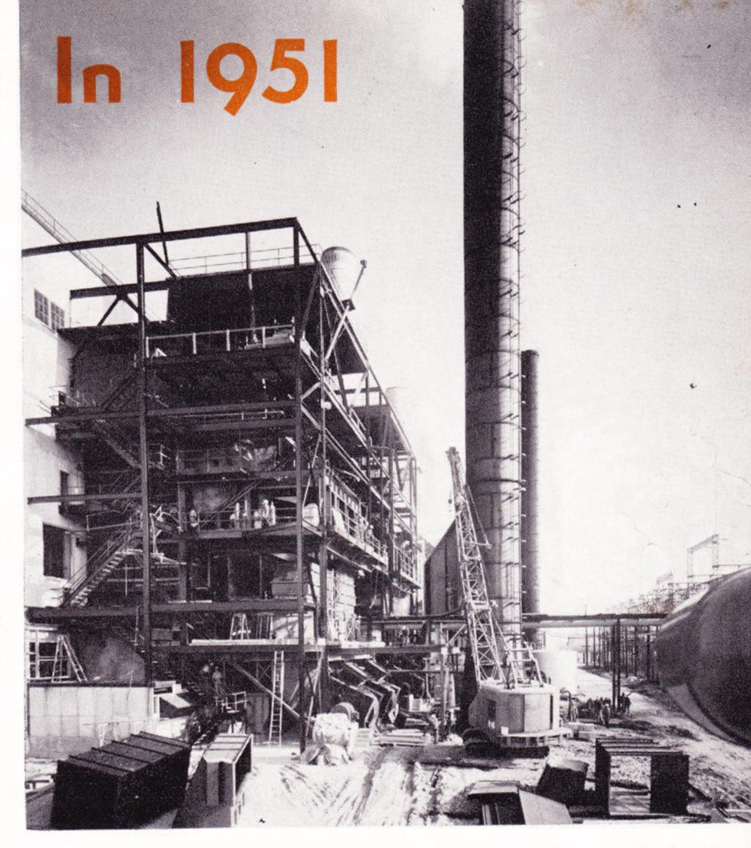
Workmen at Neches install duct work (above) for No. 6 unit's forced and induced boiler fans as others (below) build a bay for a 75,000 kva 69 kv transformer bank.
