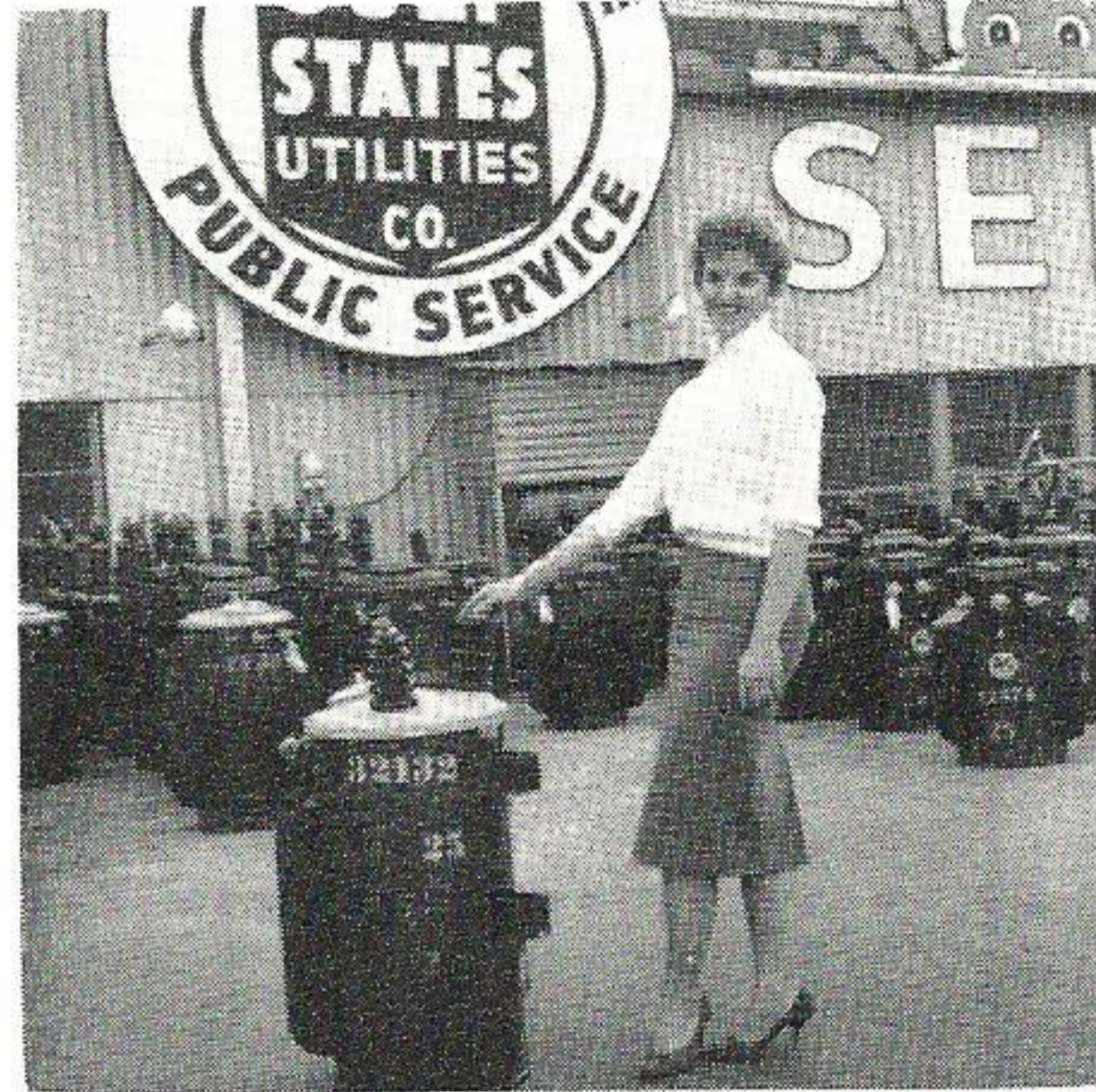
I. 25 kva distribution transformer
