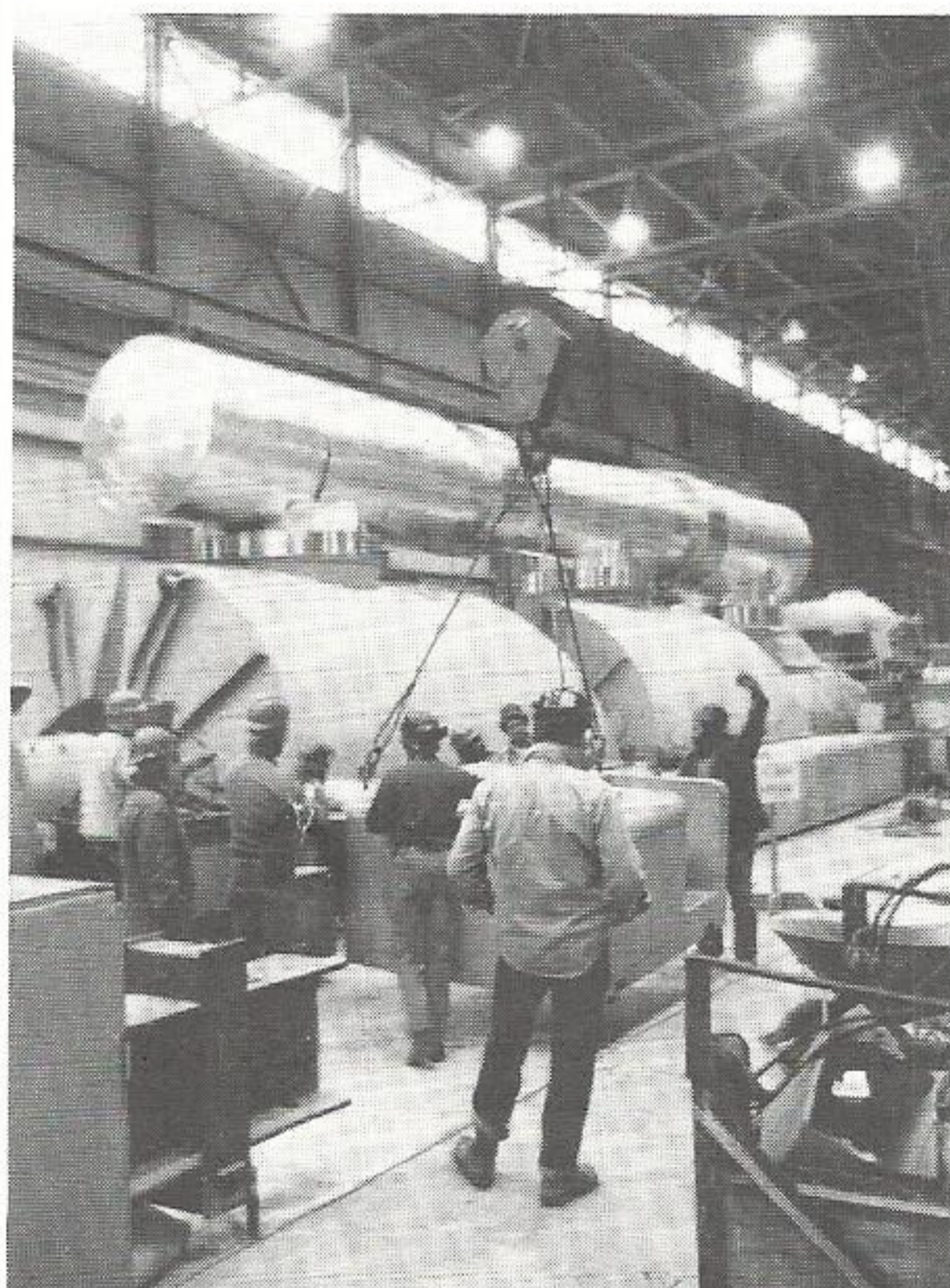
Mid-Valley employees install turbine.
