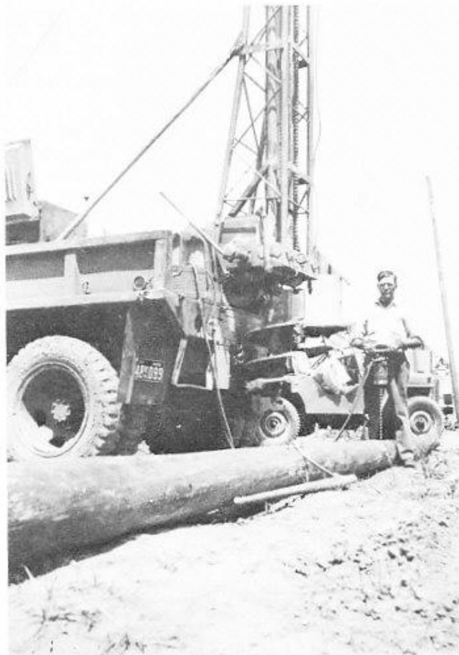
E. J. Alonzo, a utility truckdriver for the company in 1945, is using the first electric drill owned by the Baton Rouge Division. The drill was made from a 6-volt truck starter and was battery powered.
