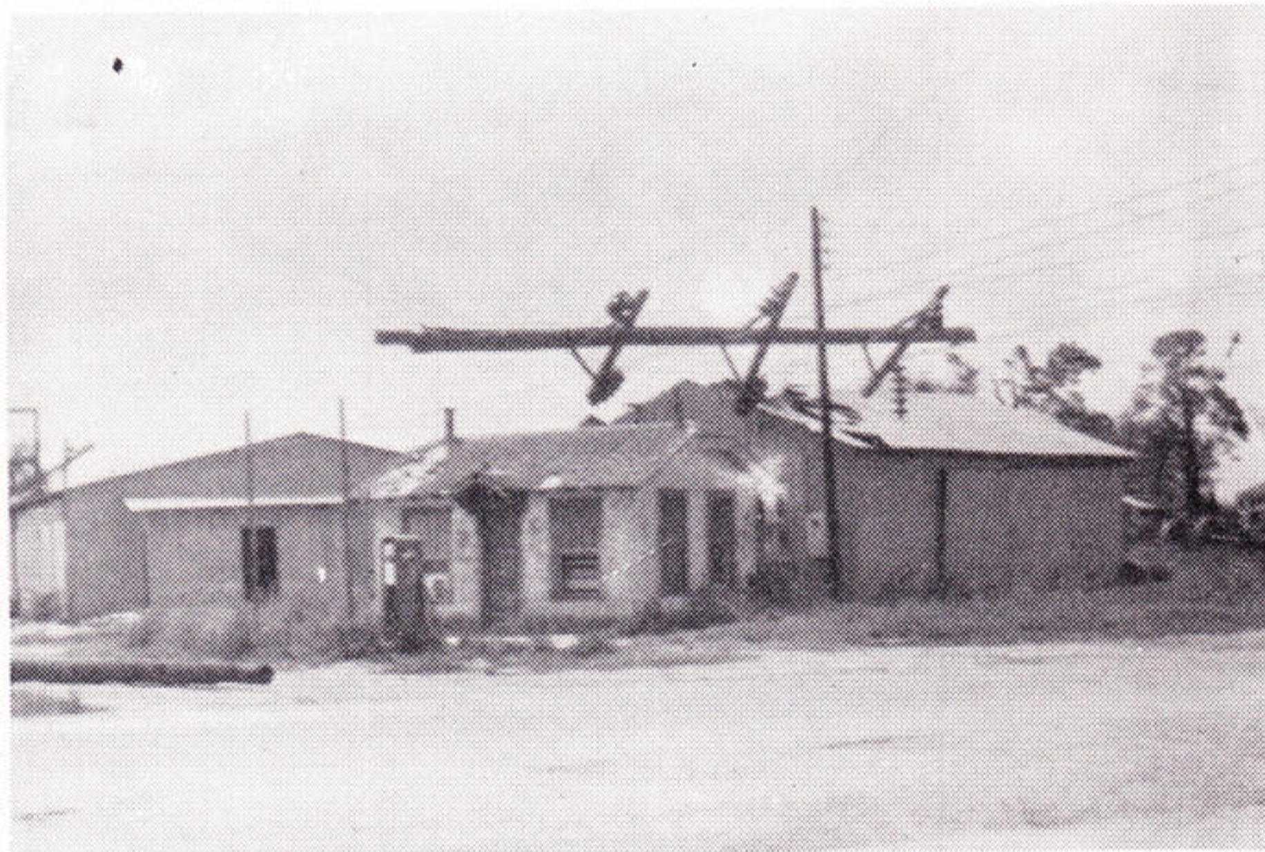
Power pole falls on garage at Roanoke, Louisiana.
