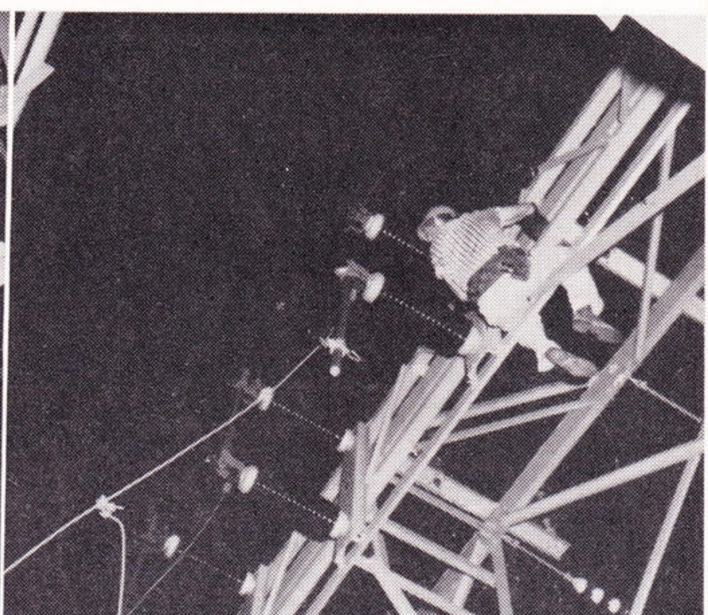
Spindletop's substation was the biggest job of the night. The large fuse in the foreground of the righthand picture had to be replaced — its circuit carried 69,000 volts.
