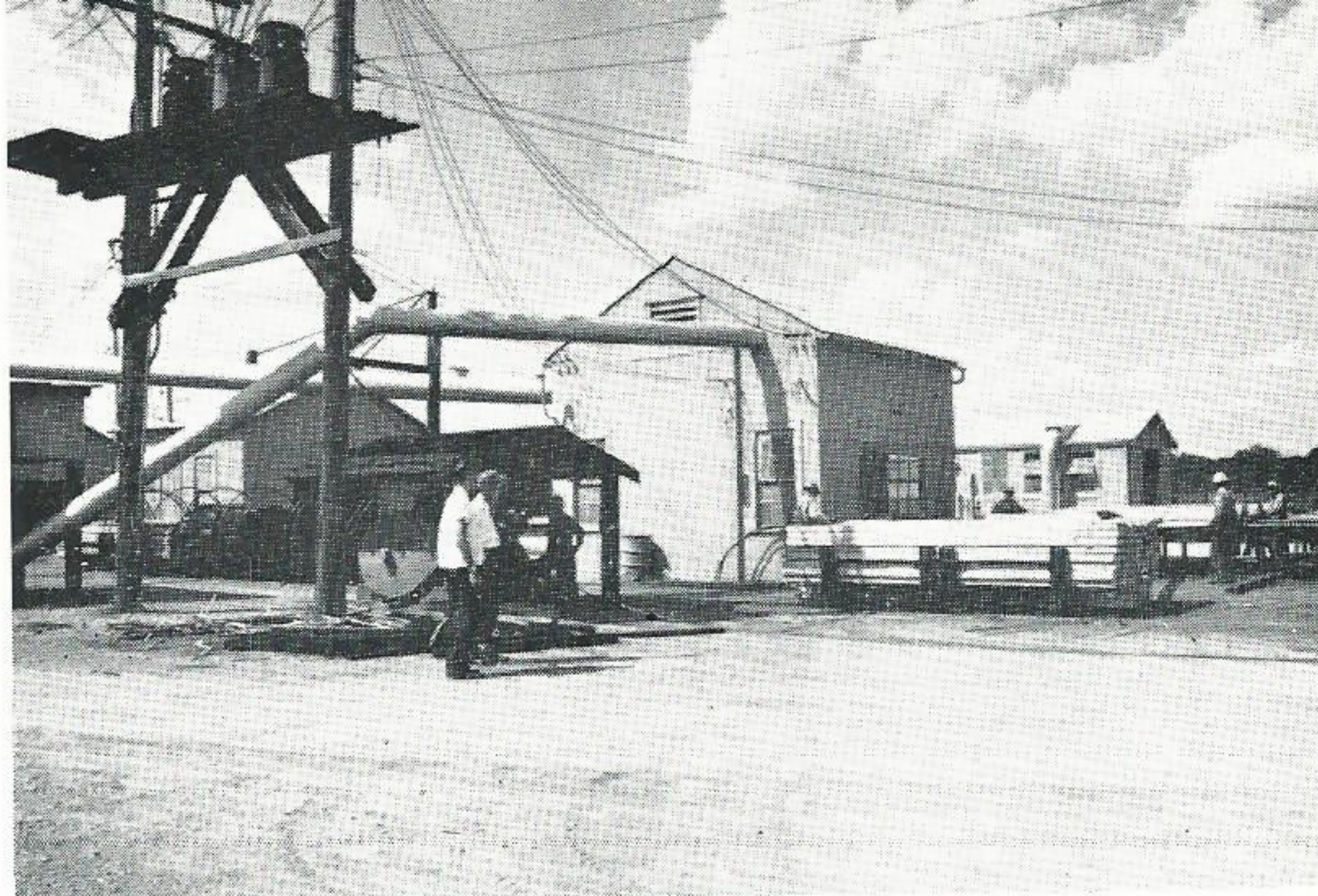
PREPARE BRIDGE TIMBERS. Workmen at the Santa Fe's tie and timber plant in Somerville manufacture and finish bridge timbers at the plant's sawmill prior to treating them with a preservative. R. C. Houston, superintendent of the plant, wearing straw hat, explains the sawmill's functions to District Serviceman Jimmy Stout.
