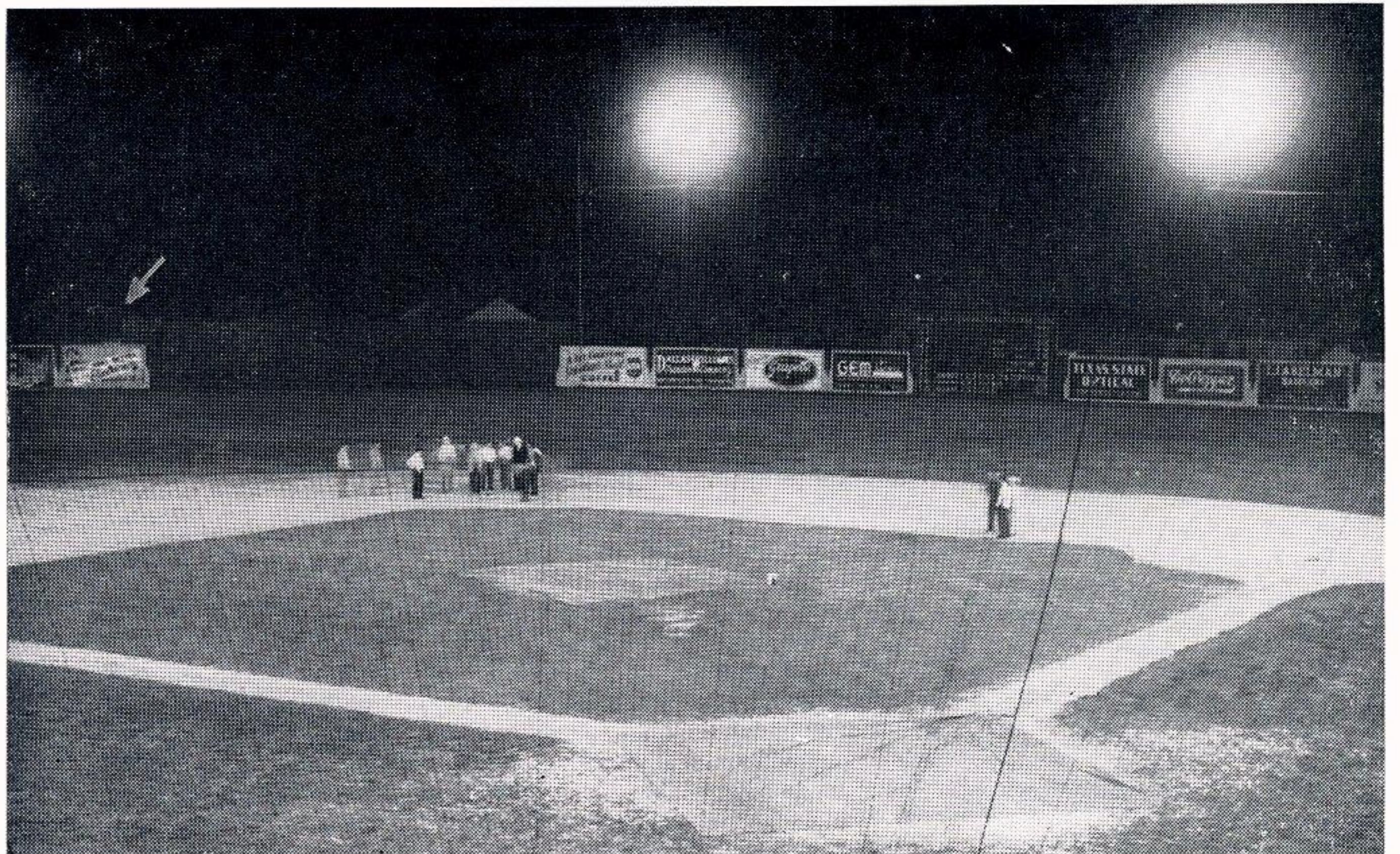
NIGHT SHOT OF STUART STADIUM UNDER LIGHTS — Just before Beaumont's opening night game officials look over the playing field to check on the efficiency of the new 378,000 watt lighting installation. Arrow points to Gulf States signboard some 450' from camera point.
