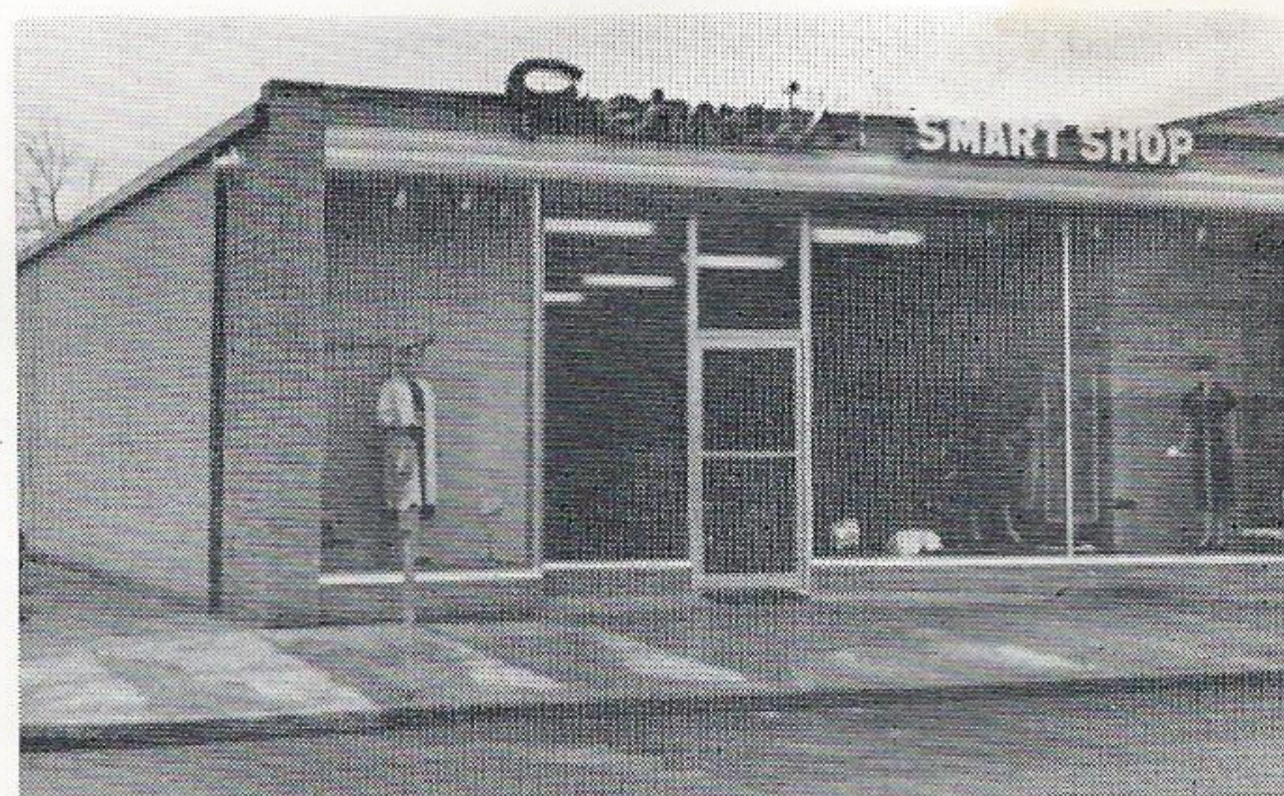
The Gervais Smart Shop is one of Jennings' newest all-electric stores.
