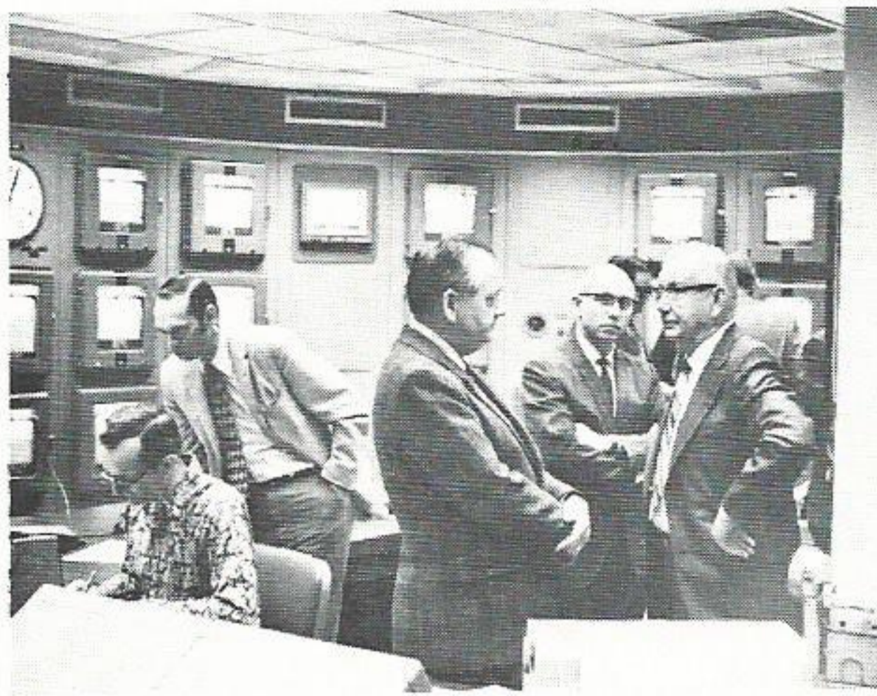
A gathering of men from the American Power Dispatchers Association, Central Area Group, were hosted by our company recently and taken on a tour of the control facility in the head office building in Beaumont. Herman Heil, seated, and Clebern Bean, right, were two of our company people on hand to help. Austin J. Mary, assistant to senior executive vice-president S. L. Adams, was the guest speaker of the meeting and spoke to the group with his speech entitled, "A Discussion of the Determination of Control Error."
