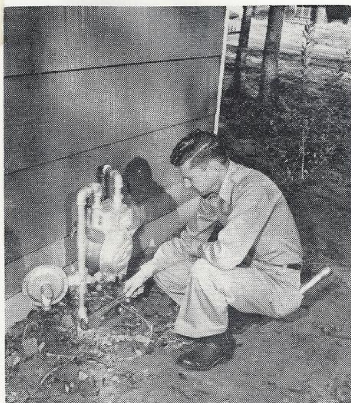
A gas serviceman's duties include installing and turning on meters . . .
