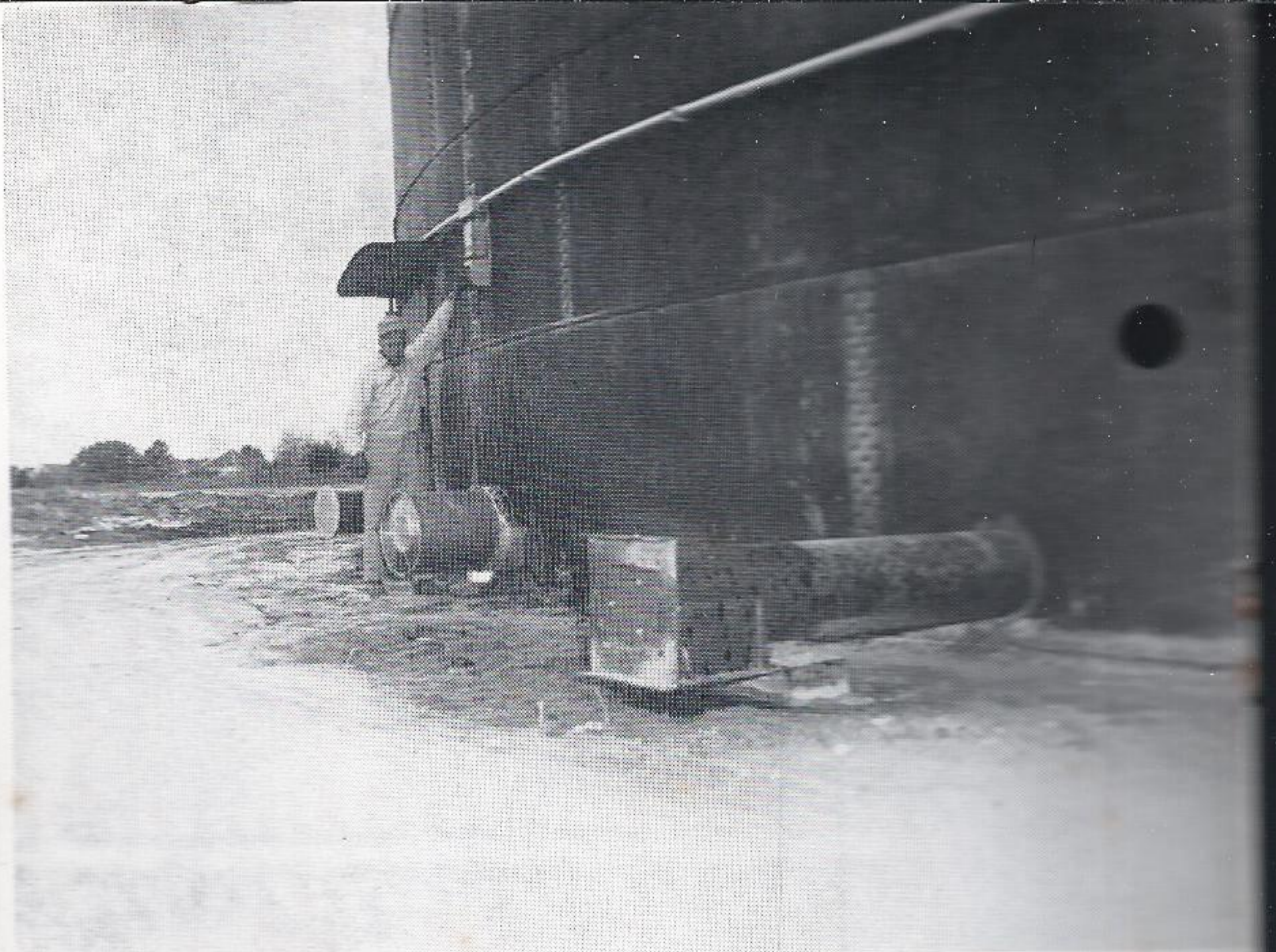
Mr. McGowan checks the vent fans. The pipe in the foreground is where the tank is unloaded by an electric auger.
