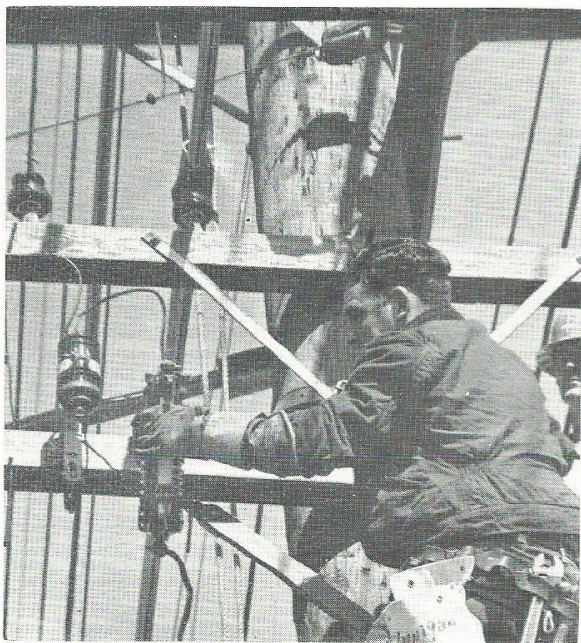
THE OLD. Here a lineman is closing a cut-out switch by hand. He feels a momentary surge of electricity. Some old timers were accustomed to this practice and took the shocks in stride.
