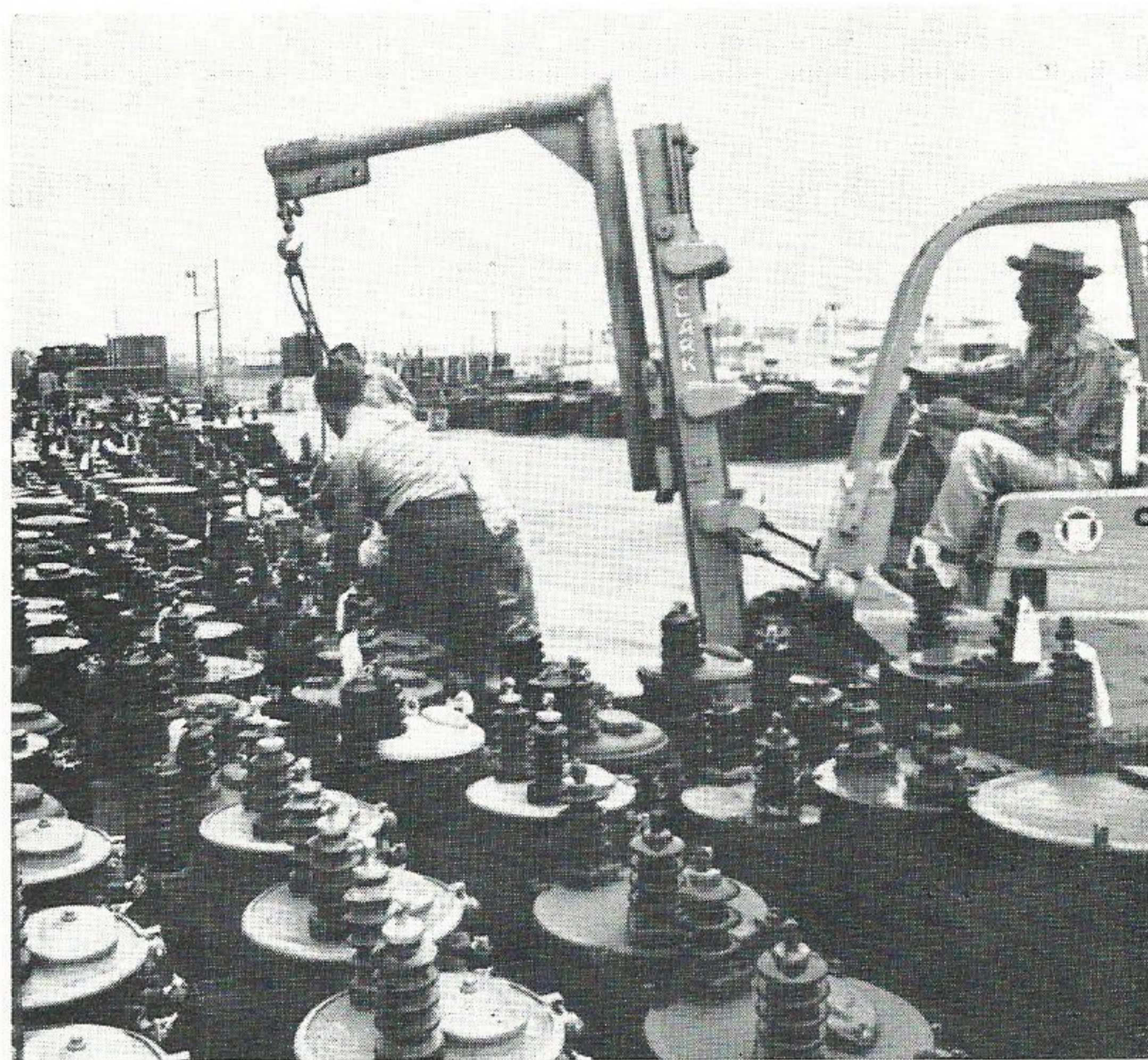
LOADING WORK. In background, John Beard selects a transformer for his job, while James Sanders in the heister hooks onto another to load it on a truck.
