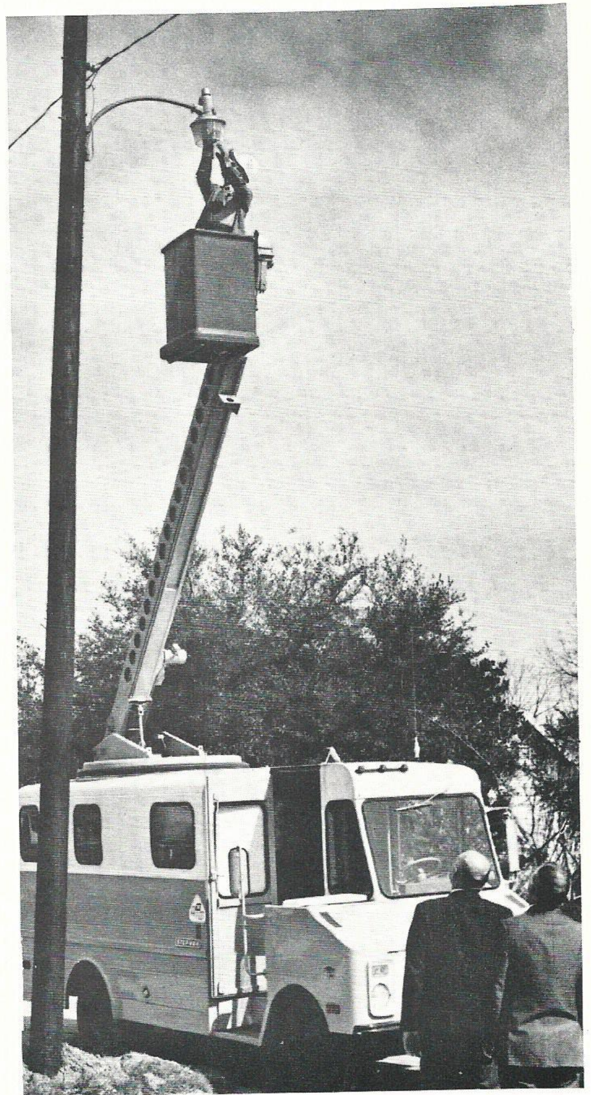
J. W. Minner, service foreman Port Arthur Division, inspects one of the new lights. The lights are built to last 24,000 hours or six years under the supervision of Mr. Minner and his men.
