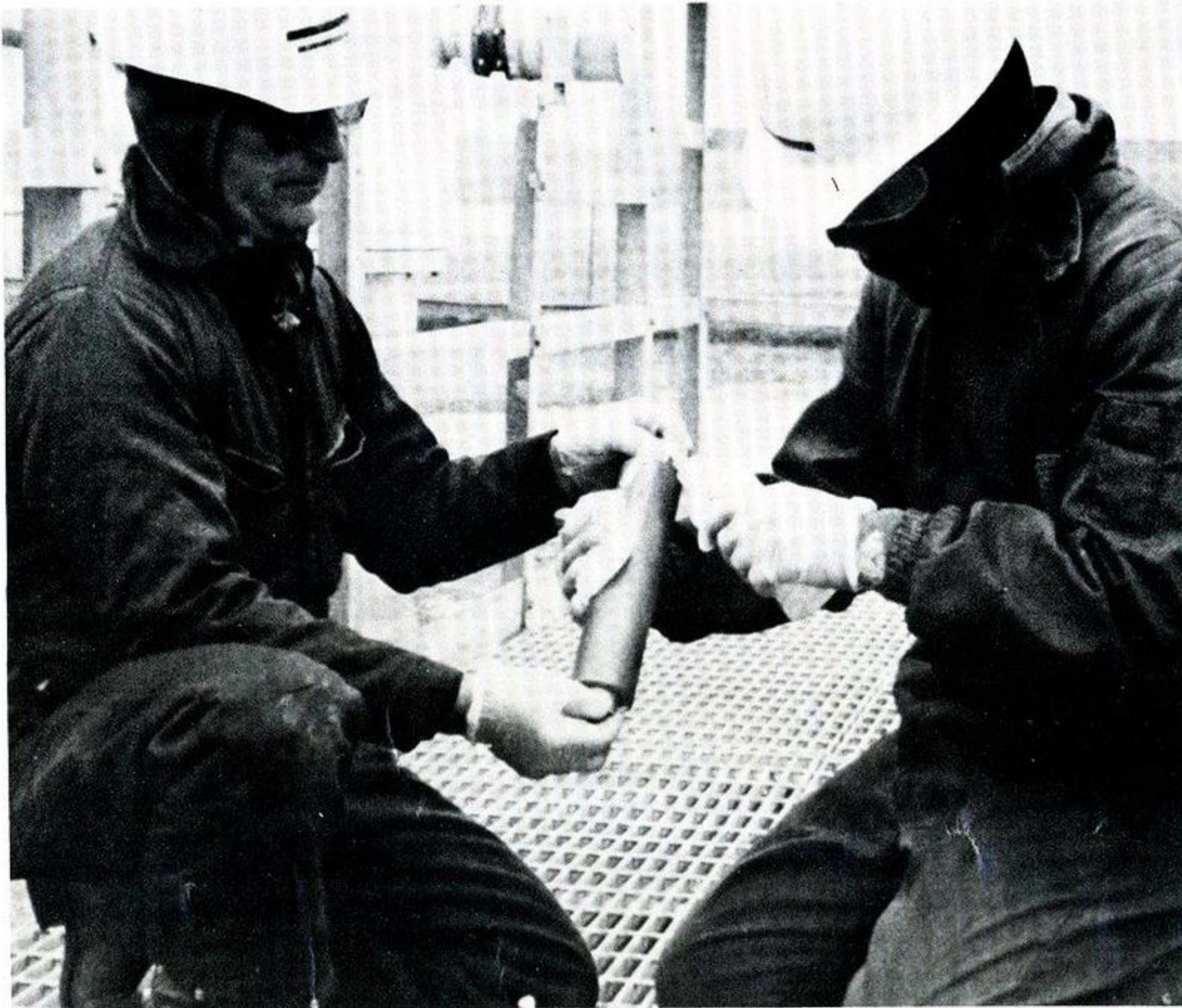
It was necessary for the gas bus at Webre to be kept immaculately clean and free of contamination during construction and much of this responsibility fell on the shoulders of the pair pictured above. Nicknamed "Mr. Clean" by co-workers, Roland Jarreau (left) and Bobby Sheets spent many hours wearing sterile surgical gloves as they went about the vital task of cleaning the gas bus equipment.
