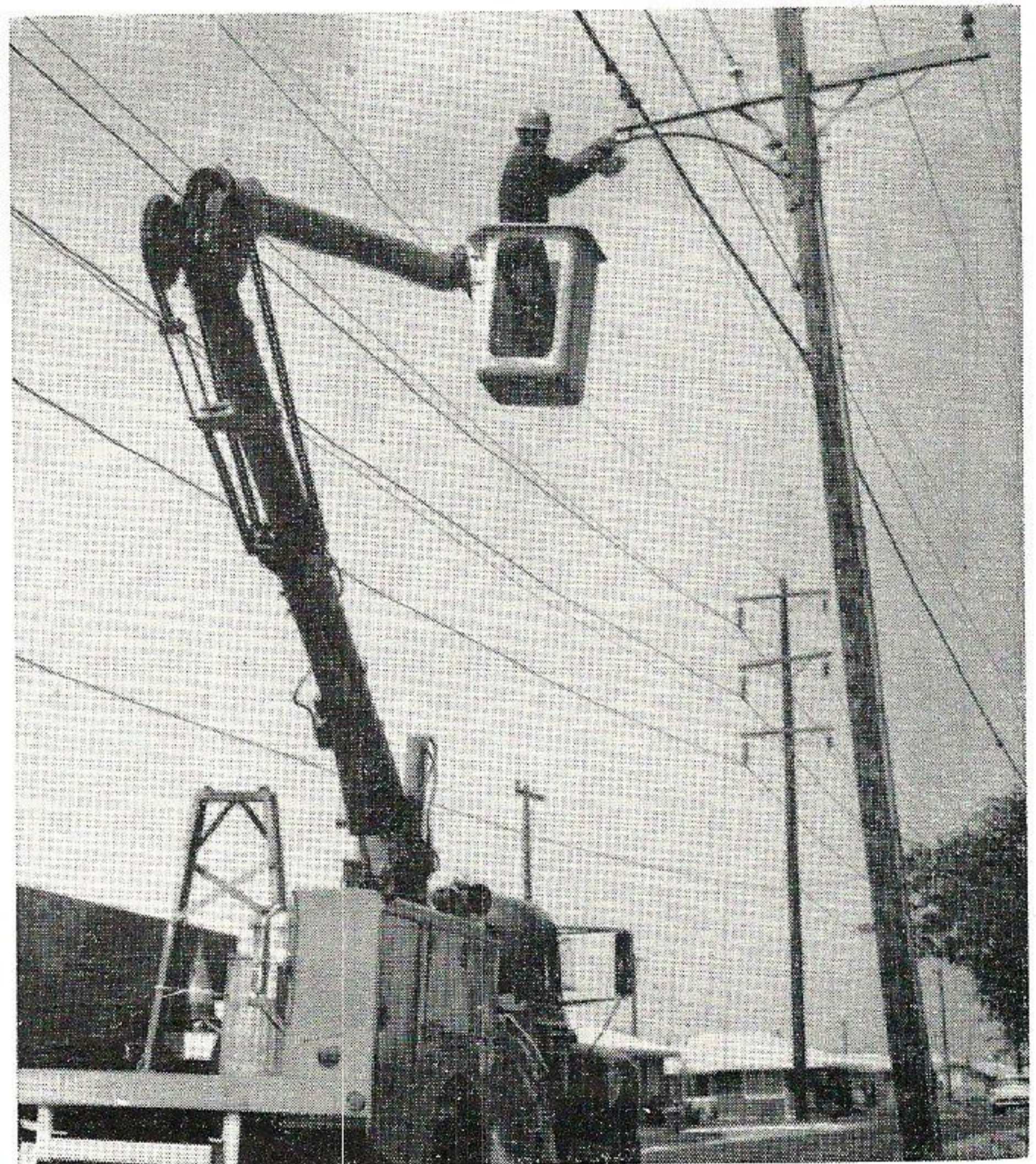
R. W. "Mac" Matulik, Line Department, Port Arthur, quickly exchanges a broken street light with the aid of the long, mobile arm of the bucket truck, which replaced the old hand cranked ladder truck.
