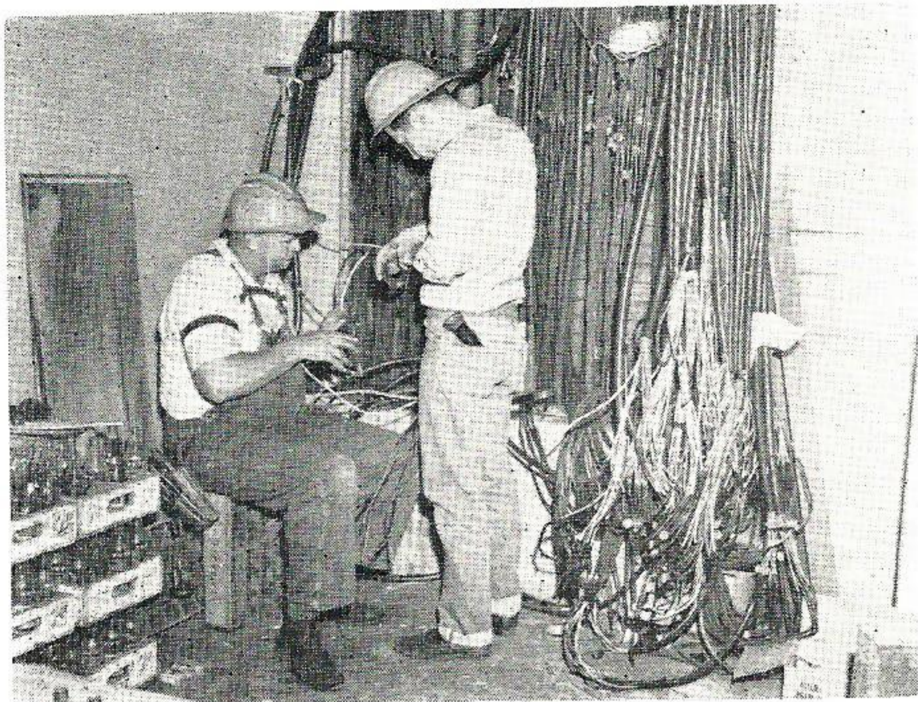
MILES OF WIRES. Two repairmen, working against the clock, reconnect some of the nerve-lines of the power plant.
