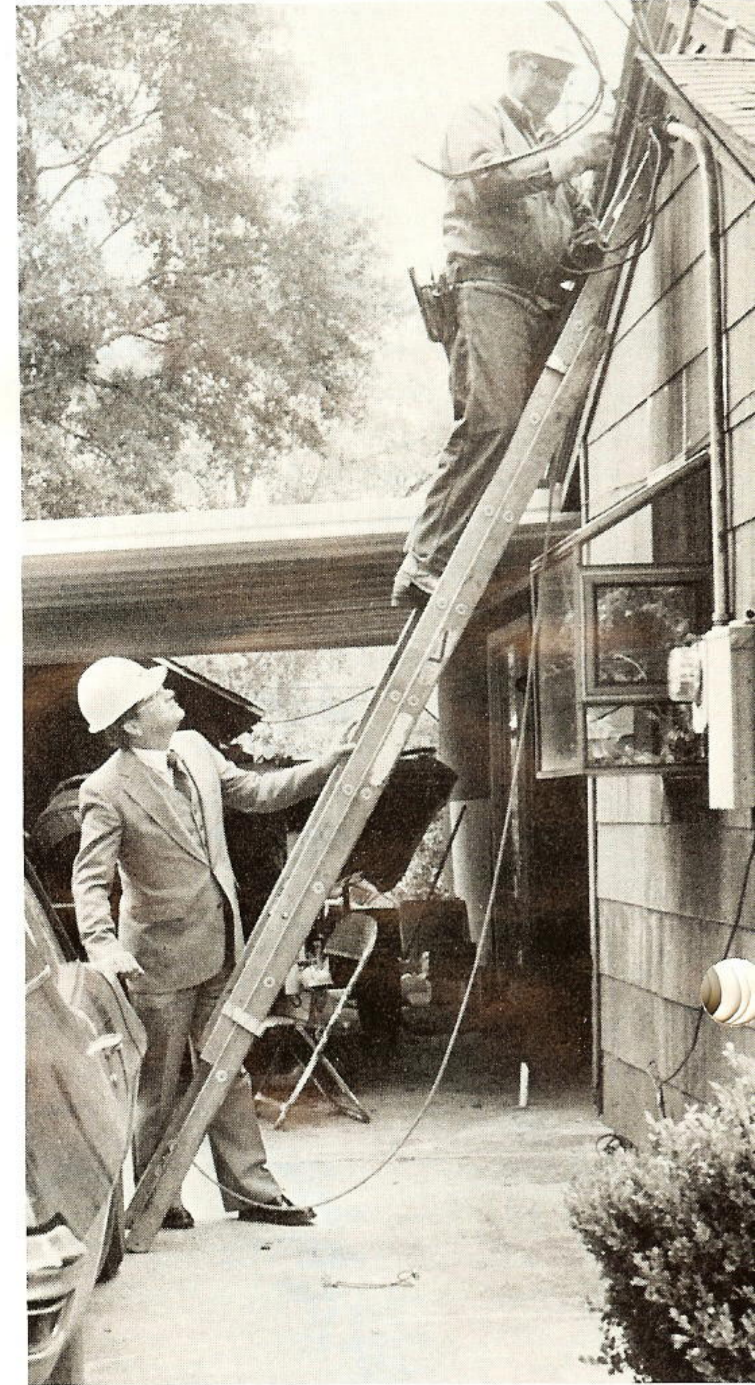
Ed Hutchins watches as Erwin Venghaus (on ladder) changes out service to a customer's ho
