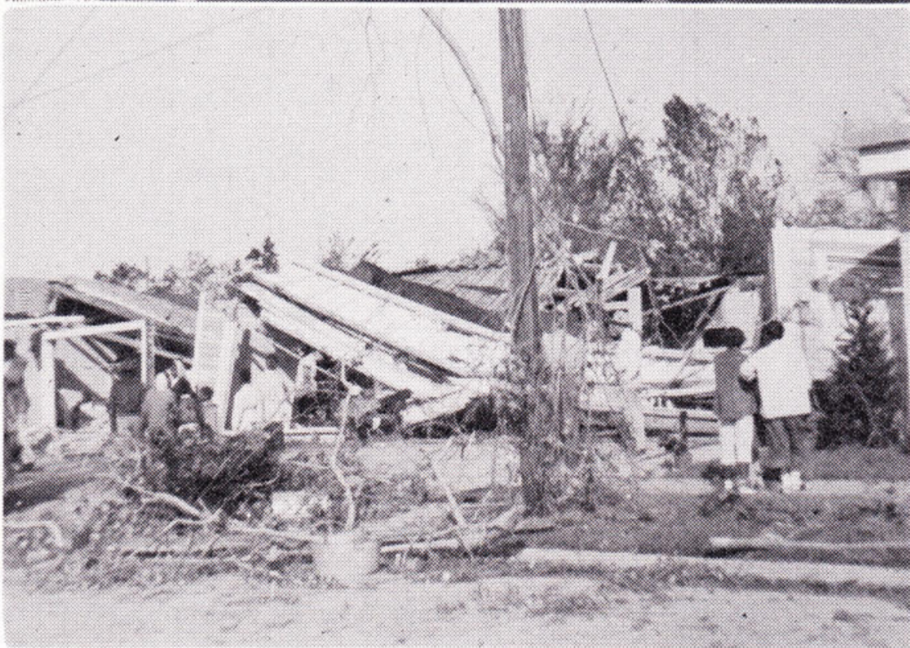
Orange felt the wrath of the tornado that swept through Southeast Texas and Southwest Louisiana this month in the Park Street area from Eighth Street to Mill Street. Gulf Staters and residents went to work to clean up debris and restore electrical power as soon as possible.
