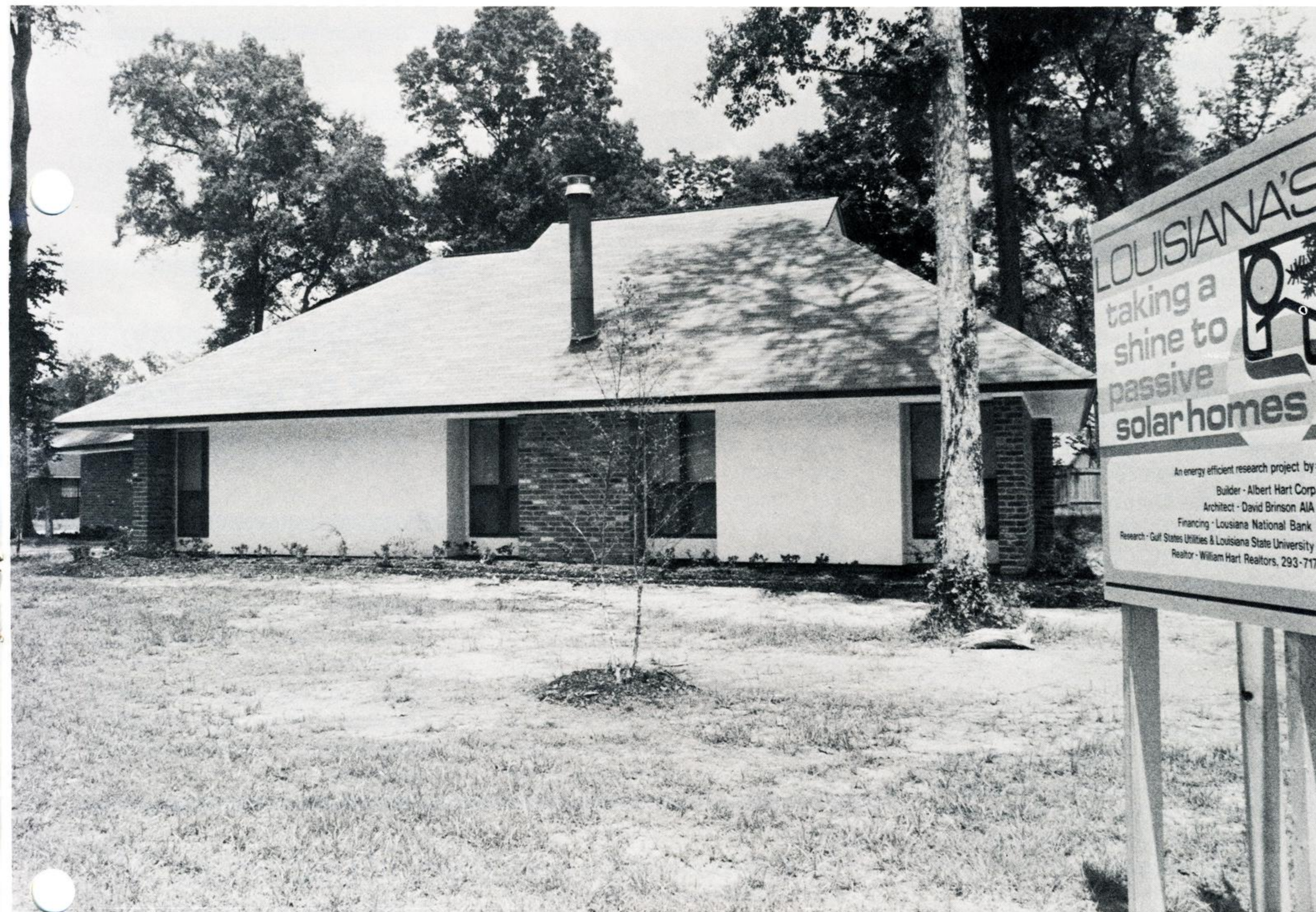
Windows are recessed to reduce radiant heat on this south-facing view.
