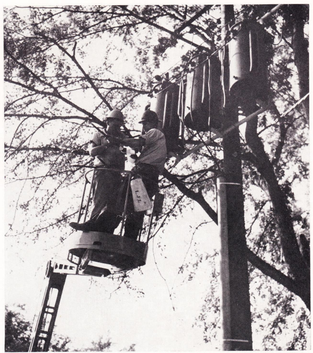
They're not picking apples, but servicemen Floyd Gonzales (left) and L. J. (Doc) Lesage are in an "apple-picker," as the hydraulic lift mounting truck is called. The picture was snappd by the "roving photographer" in Baton Rouge and appeared in the State-Times.
