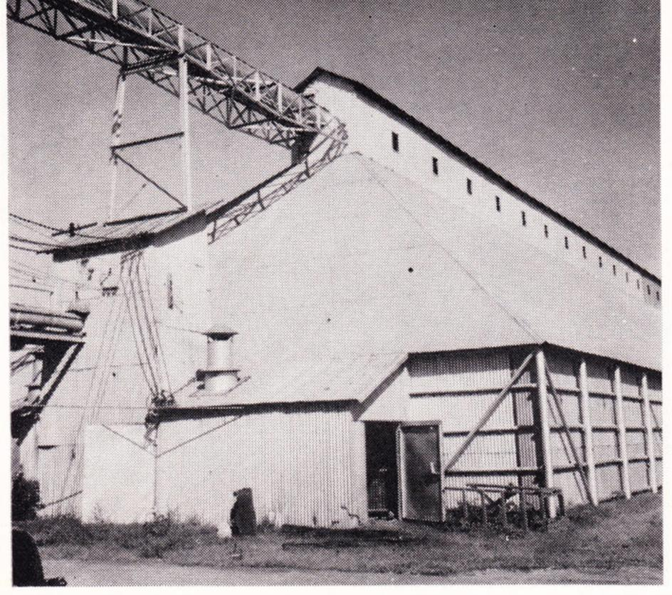
After being weighed on 50-foot platform scales, cottonseed is unloaded by air and stored in one of the company's three storage units. While awaiting processing it must be kept cool and dry by circulation of air. A single storage house may contain 7,000 to 9,000 tons of seed.
