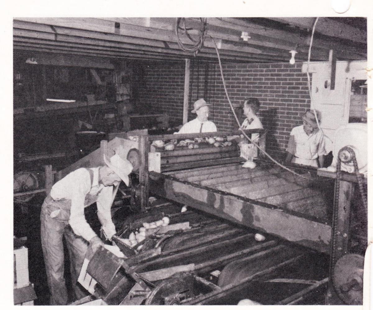
JUST outside of Church Point is Francis Bertinot's sweet potato packing plant, which was in full swing when this picture was made. Jim and Mr. Bertinot (far side of machine) watch special "sizer" or grading equipment in operation. The machine automatically separates the yams according to size and sends them into different boxes. It's Mr. Bertinot's own design.
