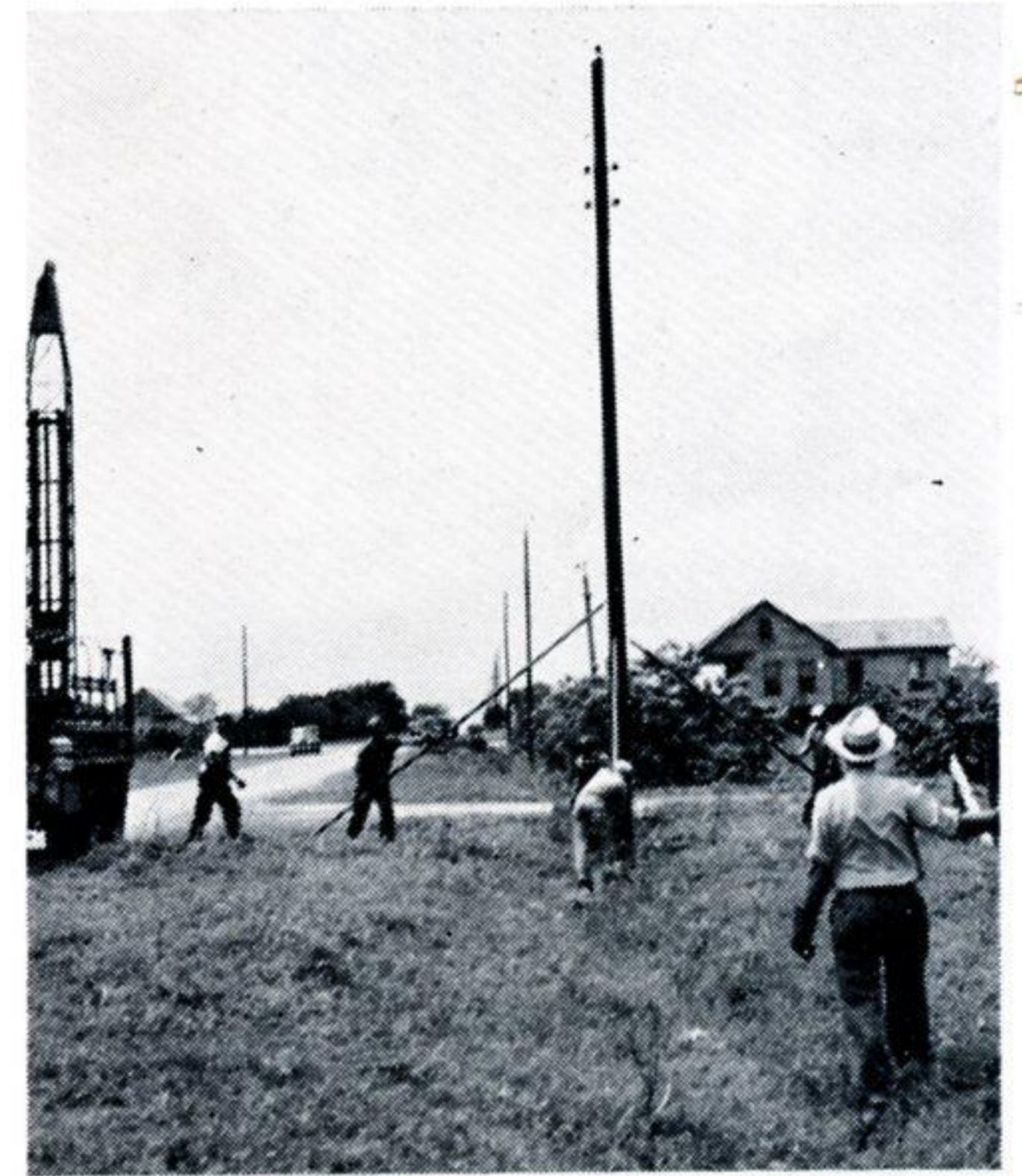
A Beaumont crew setting poles at Bolivar. The house in the background is typical of Port Bolivar homes.
