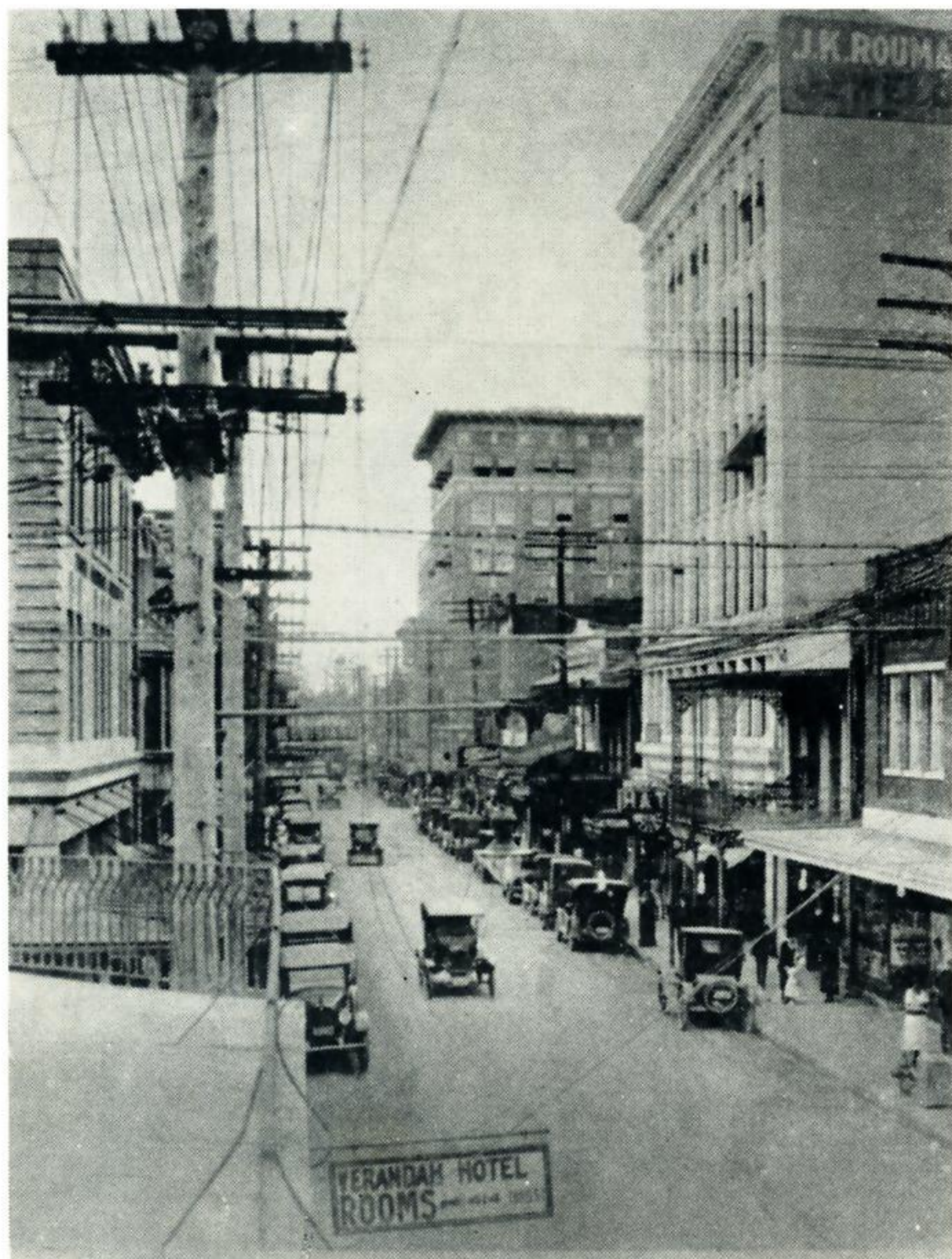
This was Third Street in Baton Rouge in 1925. Some of the old river town's wrought iron grillwork still was in evidence, and overhead electric service left a web of wires above the street.
