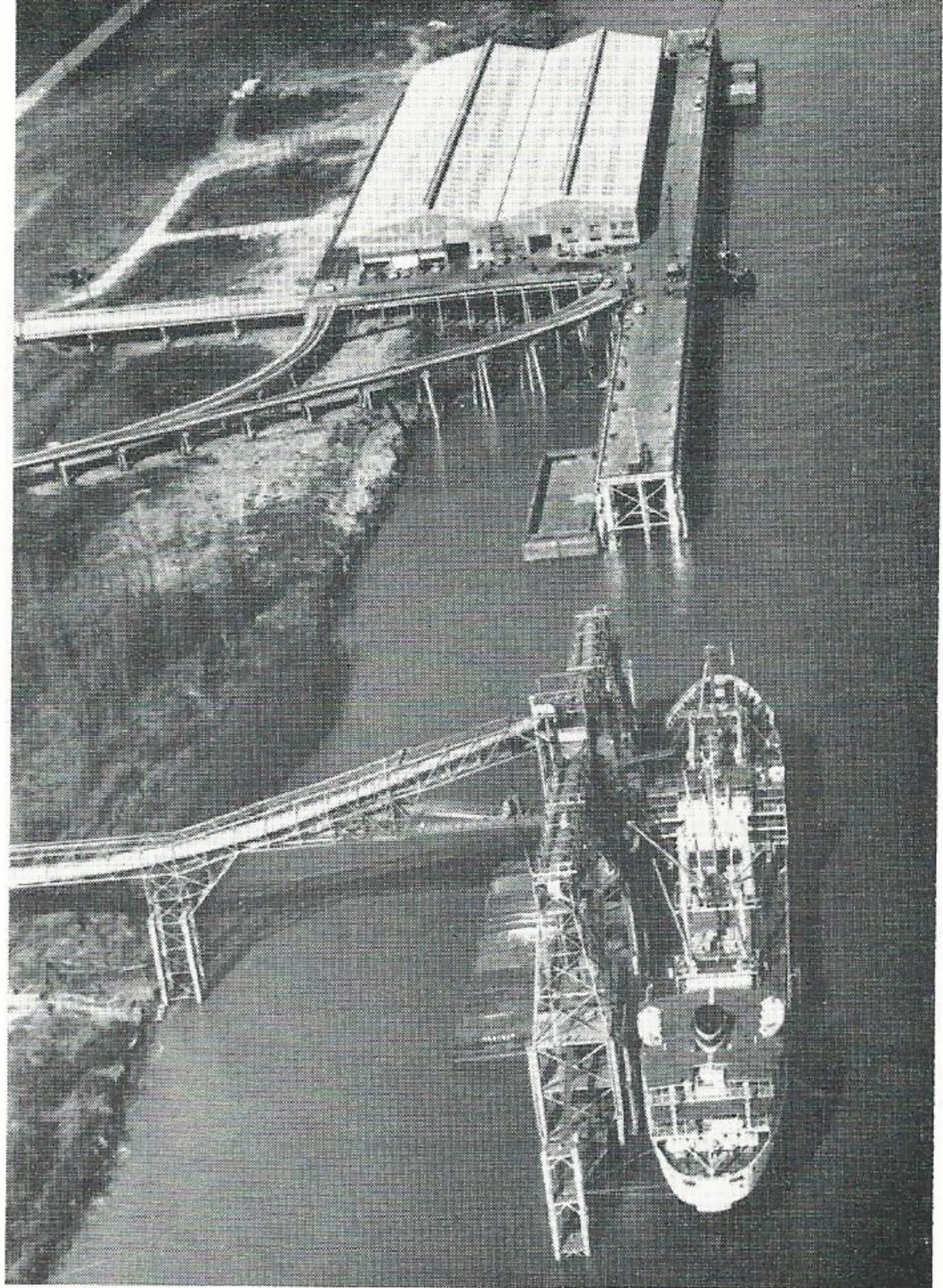
VISITOR FROM THE SEA. This ocean-going grain ship has sailed up the mighty Mississippi to the Port of Baton Rouge to take on a cargo of rice at the Port's grain docks. The grain is moved from the elevator to the grain berth by conveyor belts. In the background is the port's general cargo transit shed with its separate loading facility.
