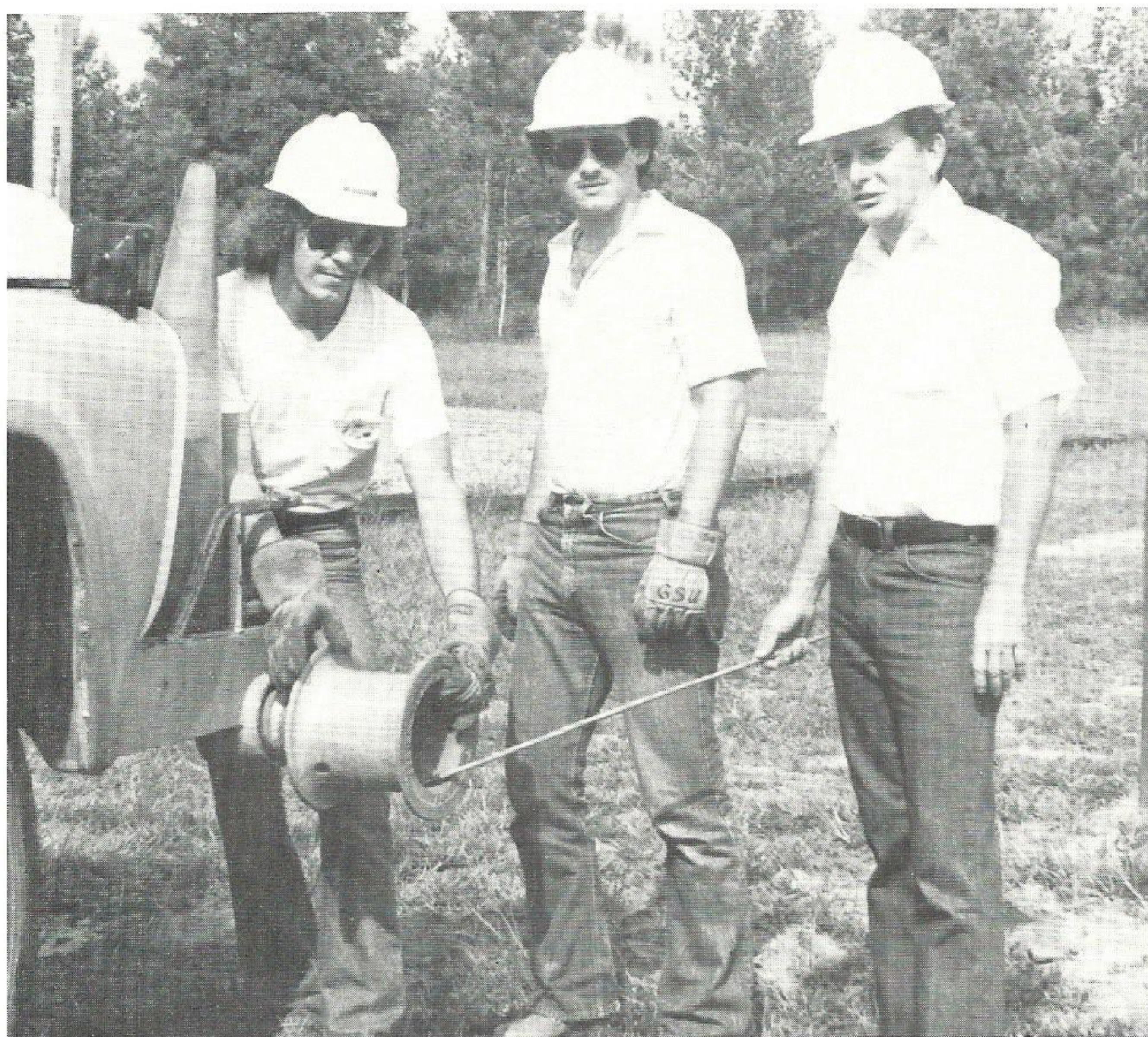
Jack Winston, mechanic-1st class of Baton Rouge, shows Steve Moore of Port Arthur (middle) and Jed Gerbrecht of Baton Rouge (left) how to install a "cat head" on a line truck. The equipment will have rope wrapped around it and then be used for dragging heavy items.
