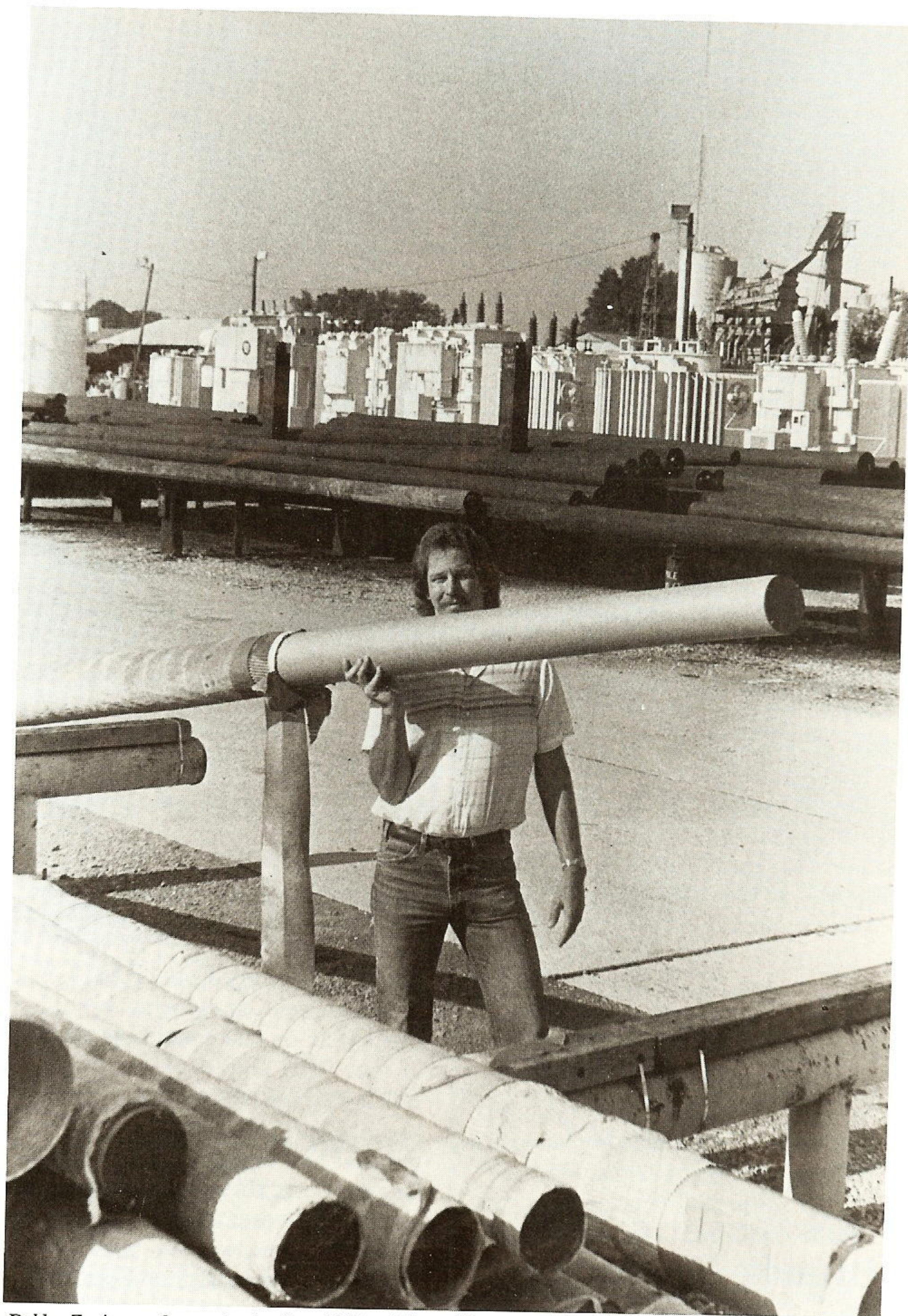
Robby Zeringue demonstrates how lightweight a fiberglass streetlight pole can be.
