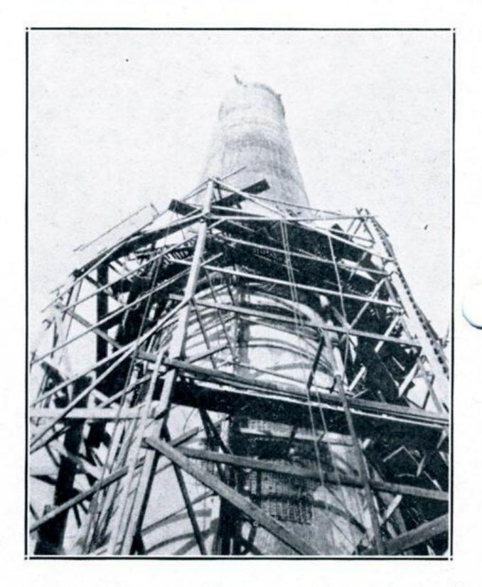
Here's an excellent wormseye view of the Lakeside station stack at Port Arthur, undergoing repairs. The entire surface is being covered with two and one-half inches of concrete, or gunnite. The cement gun method, giving 75 per cent more strength than ordinary concrete, is being used by the Cement Gun Company, under direction of the Construction Division of Stone and Webster.
