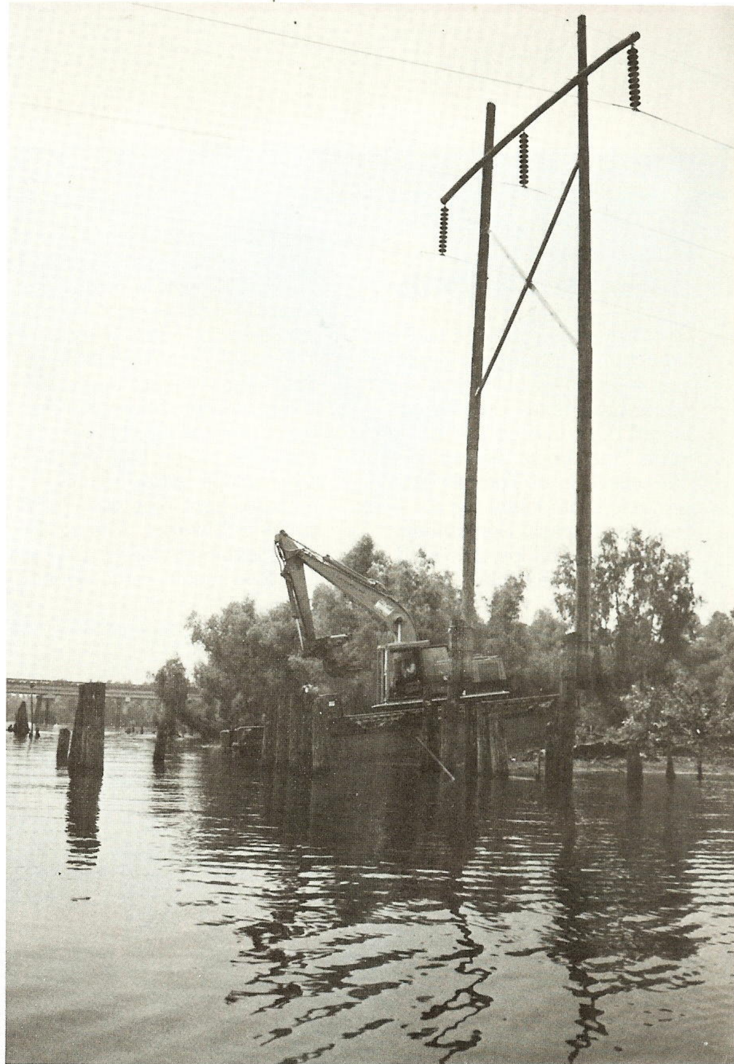
A tree-chewing tractor clears the right-of-way (above) before beginning the float to the next island (right). GSUer Mike Laborde checks progress with one of the contractors clearing for 500kv Line 760 (below).
